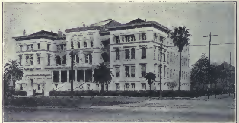
The Josephine Hutchinson Memorial Building, Headquarters for the New Orleans Session.
