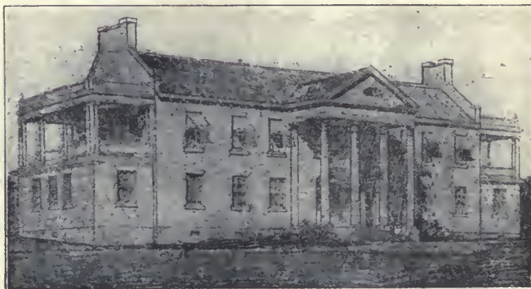
Fig. 1.—Front view of building (from architect's drawing): Exterior walls are of red brick with roof of red tile; exterior woodwork is painted white; the colonial style is especially adapted to this building, because of its prominent site and spacious grounds.
