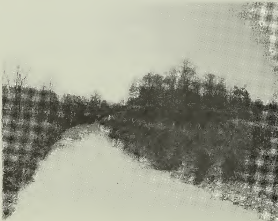
Channel work provides adequate outlets for on-farm drainage systems.
