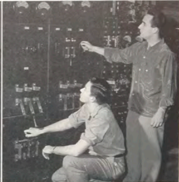
Starting auxiliary D.C. generator
