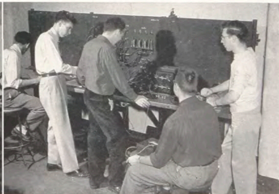
Current and power measurement in A-C resonant circuit
