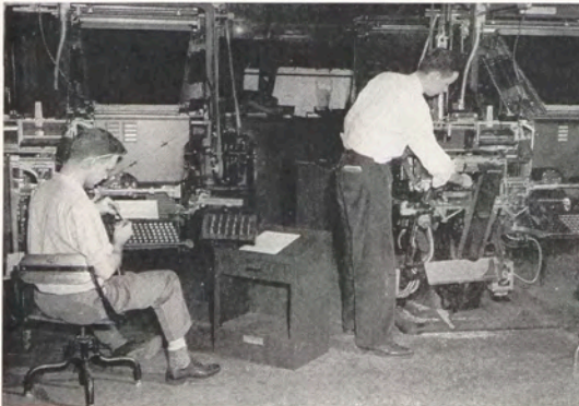
Working on the new Intertype machines
