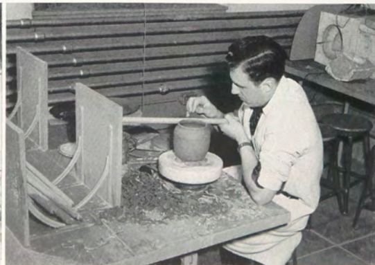
Trimming a pot in the jigger
