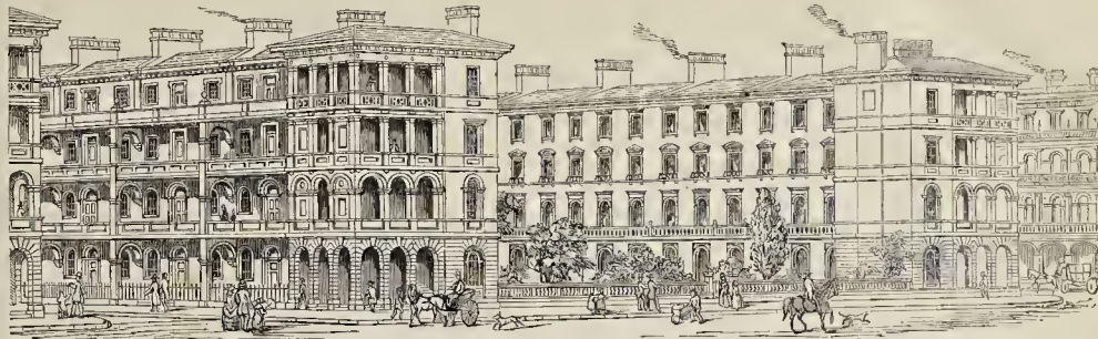
VIEW SHOWING PUBLIC STAIRCASES AND GENERAL ARRANGEMENT OF THE STREETS AND SQUARES.
