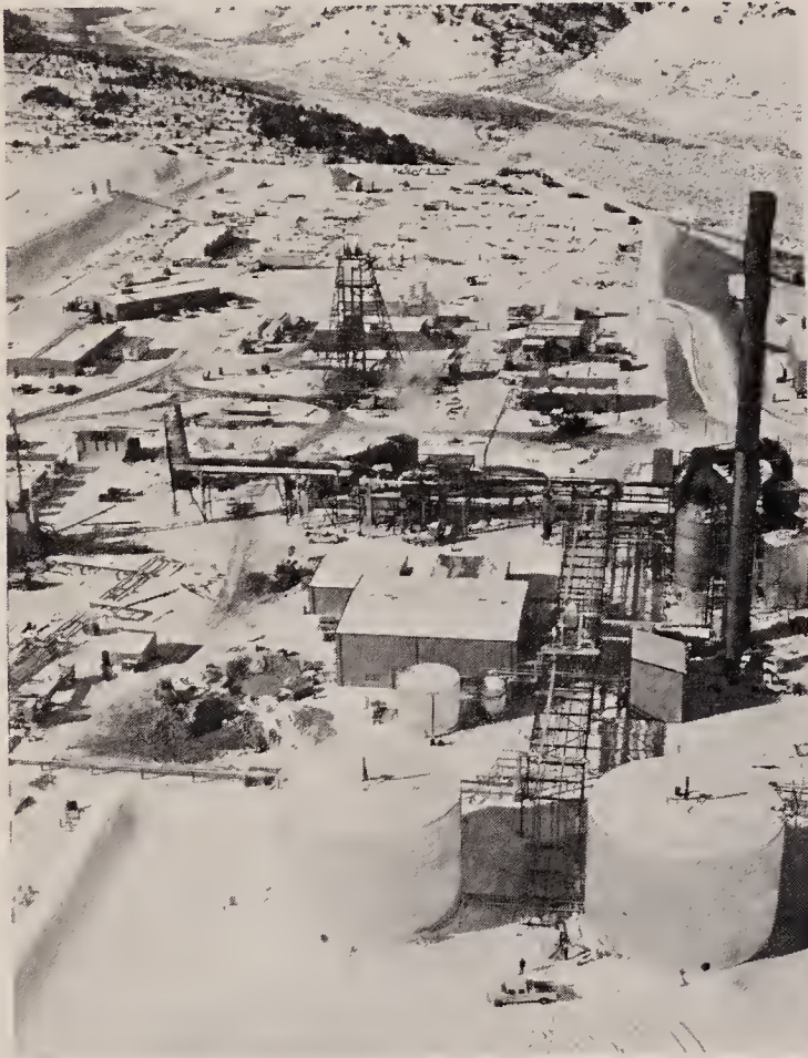
Aerial view of gas processing facilities on lease C-a.
