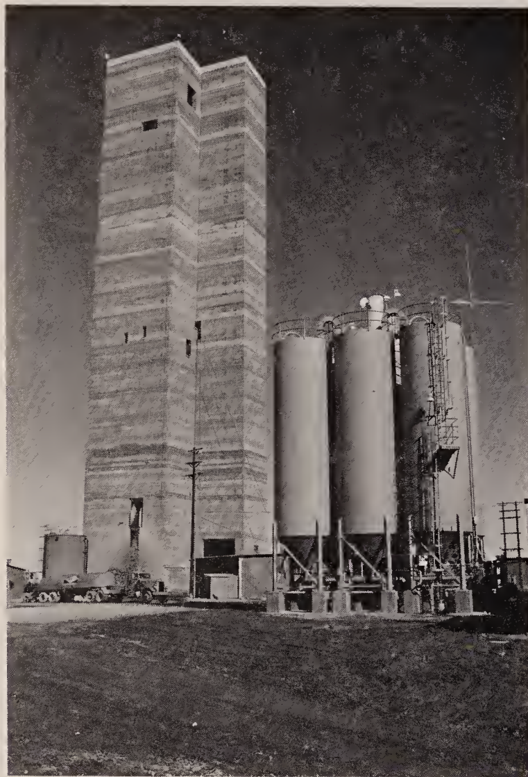
Production shaft headframe (313 feet high) and concrete storage tanks on lease C-b.
