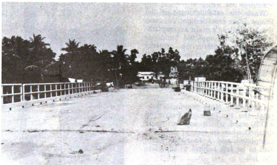
One of several bridges built in Tay Ninh by Philippine Civic Action Groups.
