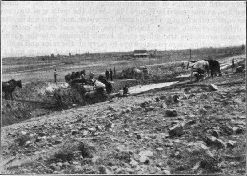
FIGURE 156.—Expensive break in irrigation ditch near Kennewick, Wash., caused by water finding its way through burrows made by pocket gophers
