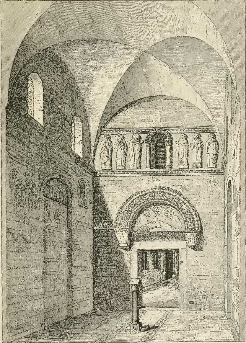
FIG. 19.—Oratory of the ancient Benedictine Monastery at Cividale in Friuli. A Lombard structure of the Eighth Century, ascribed to Gertrude, Duchess of Friuli. (From Gailhabaud.)
