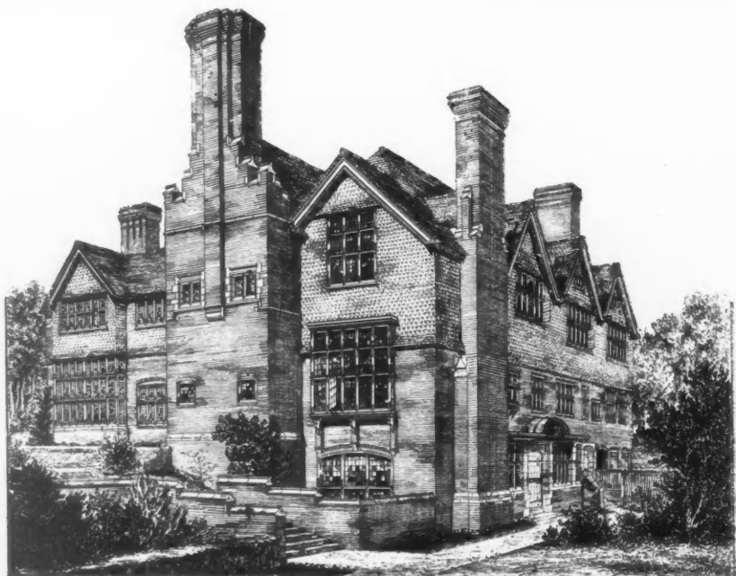
Residence for Frank Holl, Esq., R.A., R. NORMAN SHAW, R.A., Architect. Froggnall Priory,
