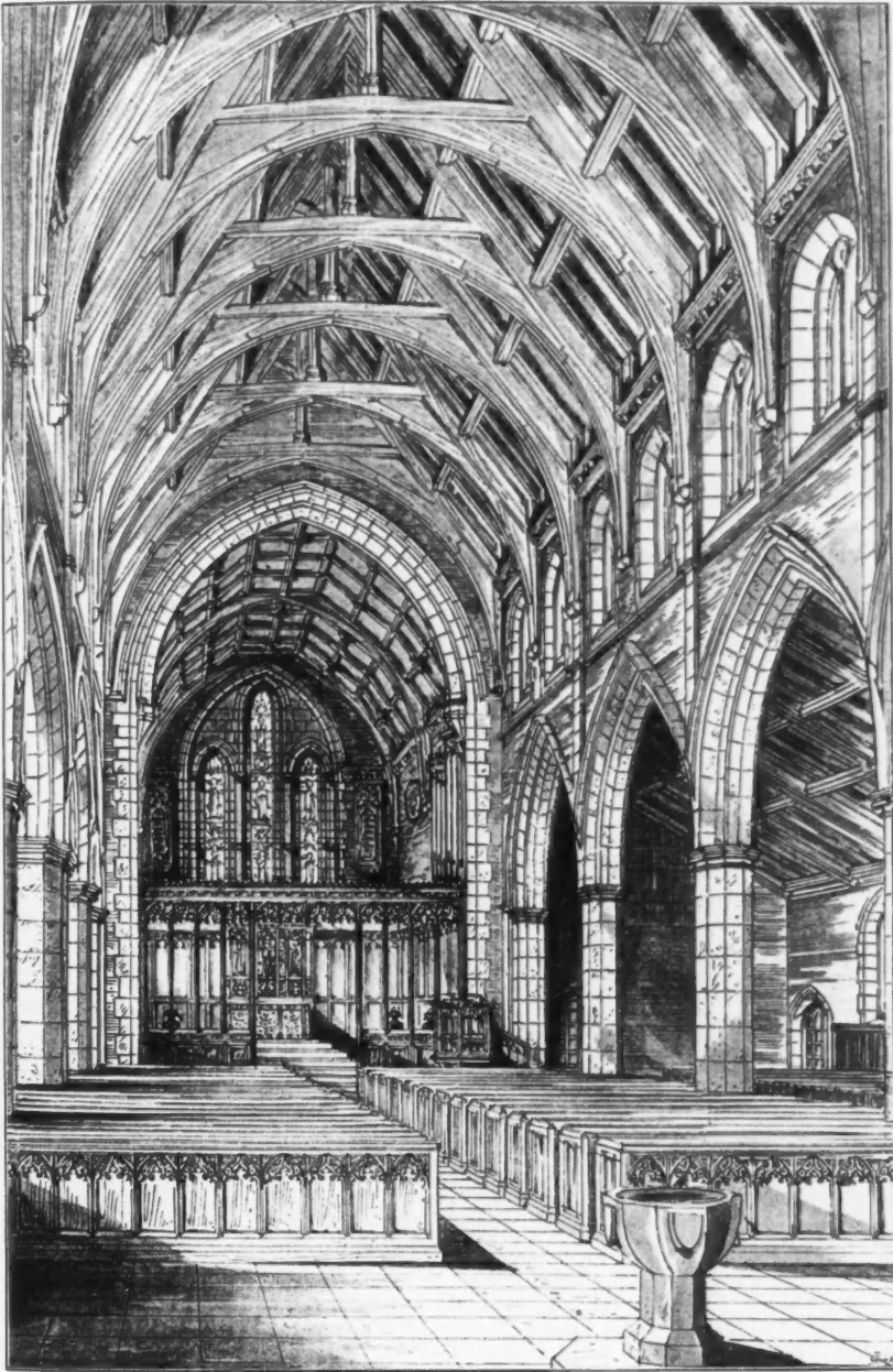
St. Hilda's Church, Sunderland, Interior, MONTGOMERY AND CARR, Architects.
