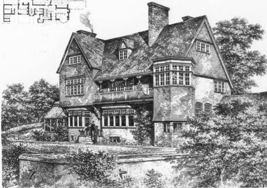
"The Kulm," Bearstead, Kent, for Dr. M. A. Adams, J. LANGHAM, Architect.
