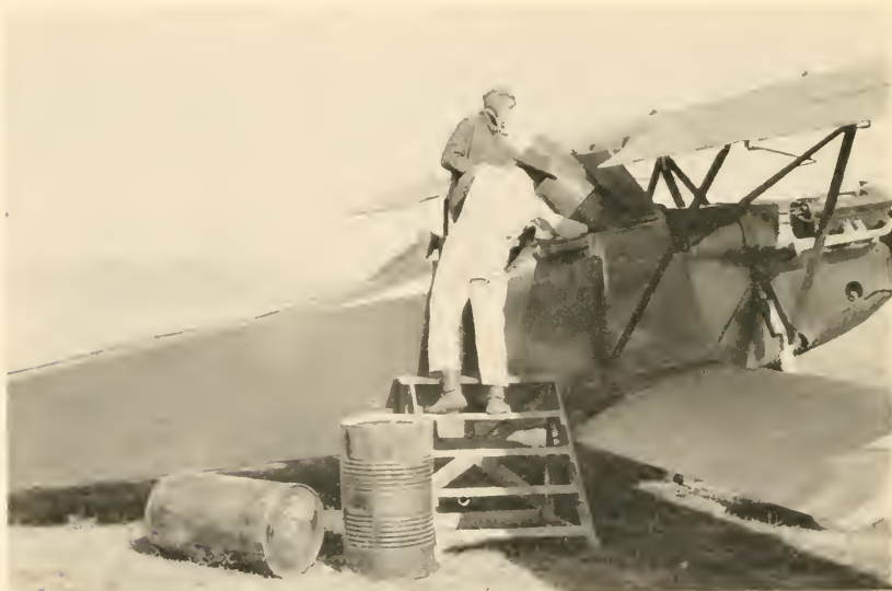
2. FILLING THE HOPPER OF AN AIRPLANE WITH CALCIUM ARSENATE. Planes carry from 300 to 500 pounds of insecticide.
