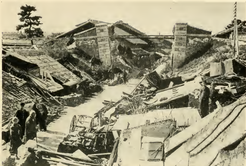
1. DAMAGE IN SUBURB OF NAGOYA, MINO-OWARI EARTHQUAKE OF 1891. (After Kikuchi.)
