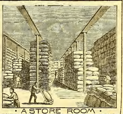
A STORE ROOM
