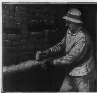
Showing row with which Plibrico is laid in place.
