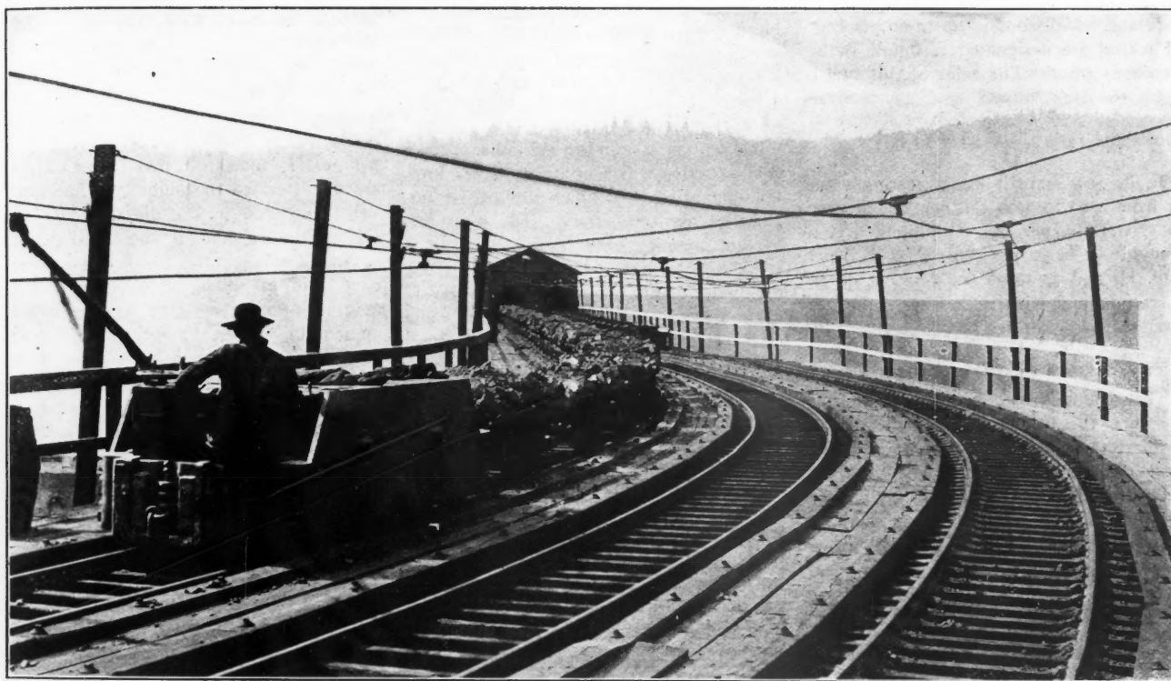
TIPPLE APPROACH TO TYLER WASHERY OF POWHATAN COAL AND COKE COMPANY
