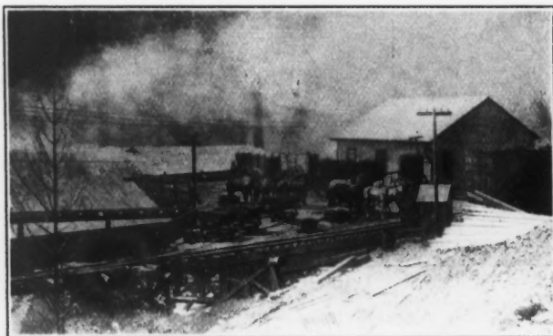
UNLOADING COKE INTO BINS
