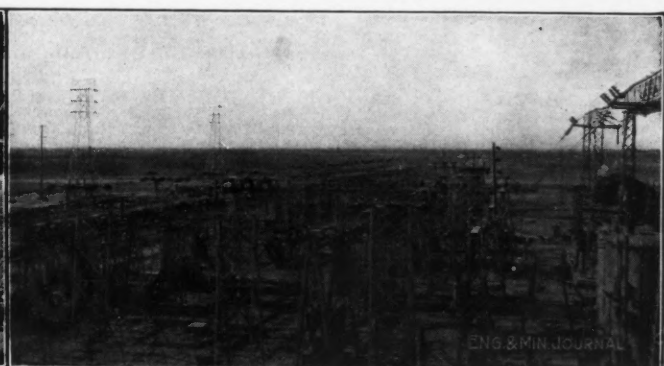
DISTRIBUTING STATION, UTAH LIGHT AND POWER CO.
