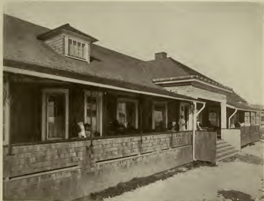
FIG. 2. LOOMIS SANATORIUM, SULLIVAN COUNTY, NEW YORK. PORCH OF OLD INFIRMARY
