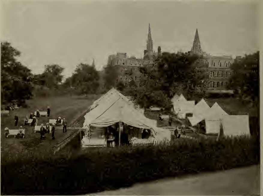
FIG. 1. MANHATTAN STATE HOSPITAL, EAST, WARD'S ISLAND, NEW YORK CITY. TENTS FOR THE TUBERCULOUS INSANE
