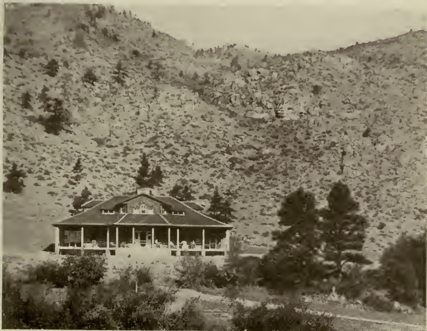
FIG. 2. ESTES PARK, COLORADO. IDEAL SUMMER RESIDENCE, WITH SPACIOUS PORCHES FOR PULMONARY INVALIDS. SLOPING GROUND, SANDY SOIL, MOUNTAINOUS BACK-GROUND AFFORDING PROTECTION FROM WIND AND DUST.
