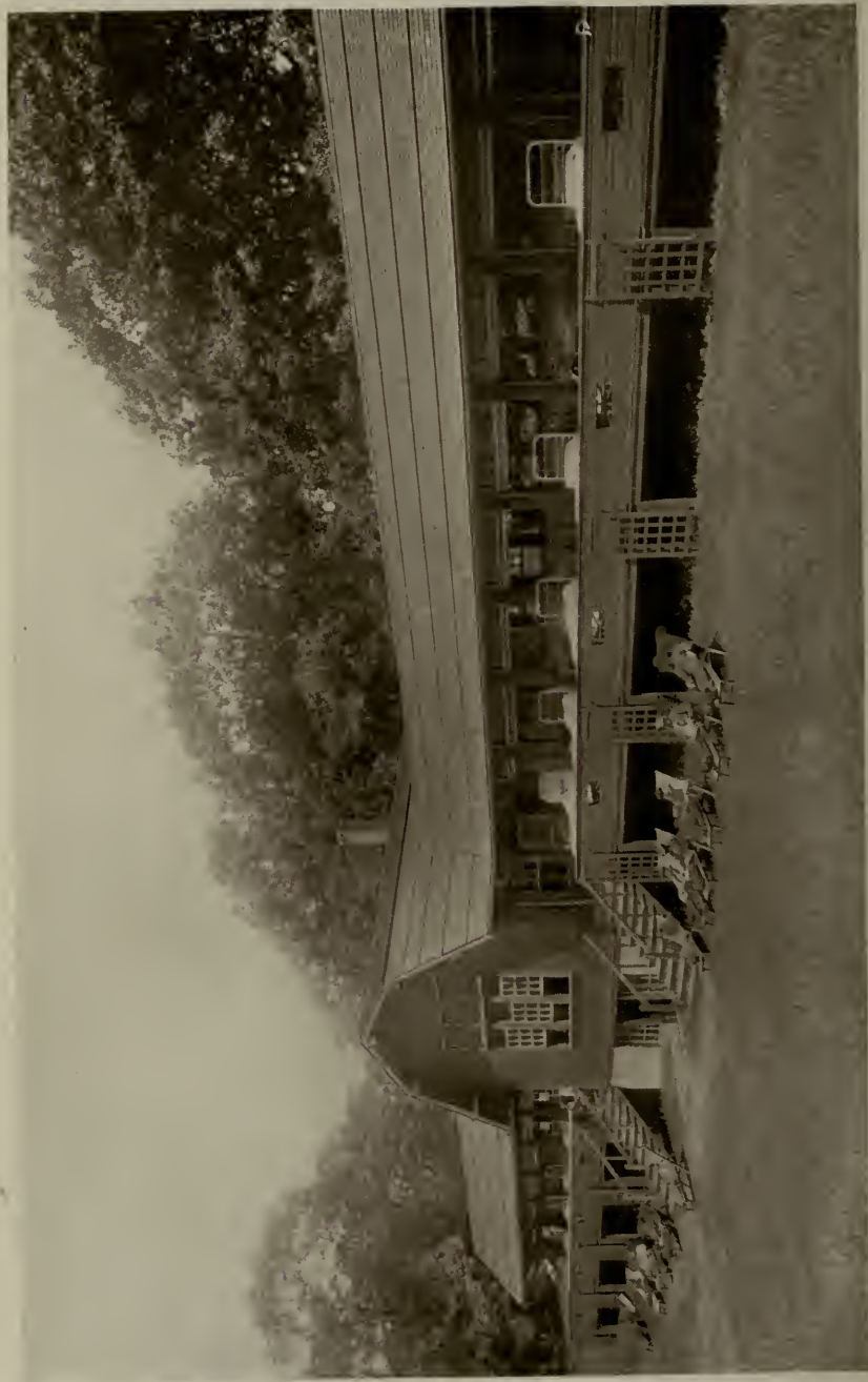
BOSTON CONSUMPTIVES' HOSPITAL AT MATTAPAN. COTTAGE WARD; LENGTH 150 FEET; CAPACITY 26 BEDS. IT AFFORDS CARE AT NIGHT FOR AMBULATORY CASES
