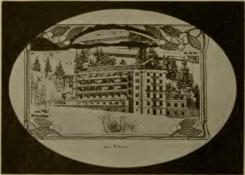
FIG. 1.—“Les Frênes,” one of the buildings at Leysin, showing balconies facing the south.
