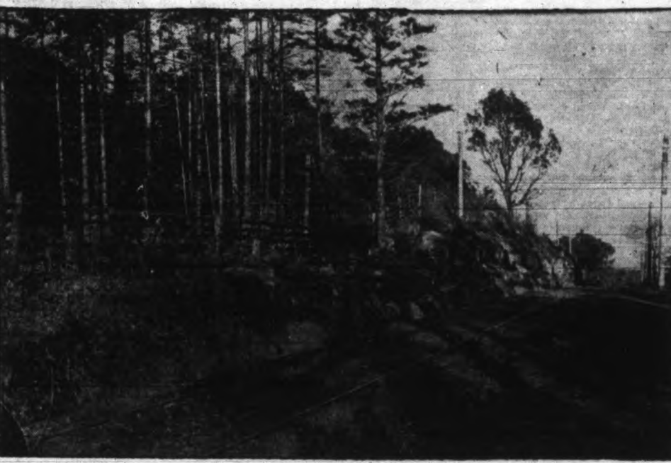
Rock Cut on Route of New Line Near Ross Bay.
