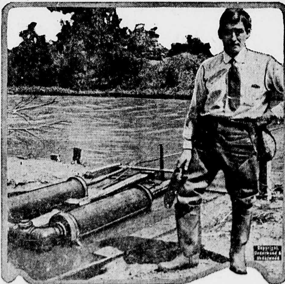
F. L. Gilman of Los Angeles, and his wonderful water pumping plant. This new motor, anchored in midstream sways back and forth, operating the two pistons shown in the photograph. It pumps 80 gallons of water a minute, and will make it possible to irrigate thousands of acres of land now arid.
