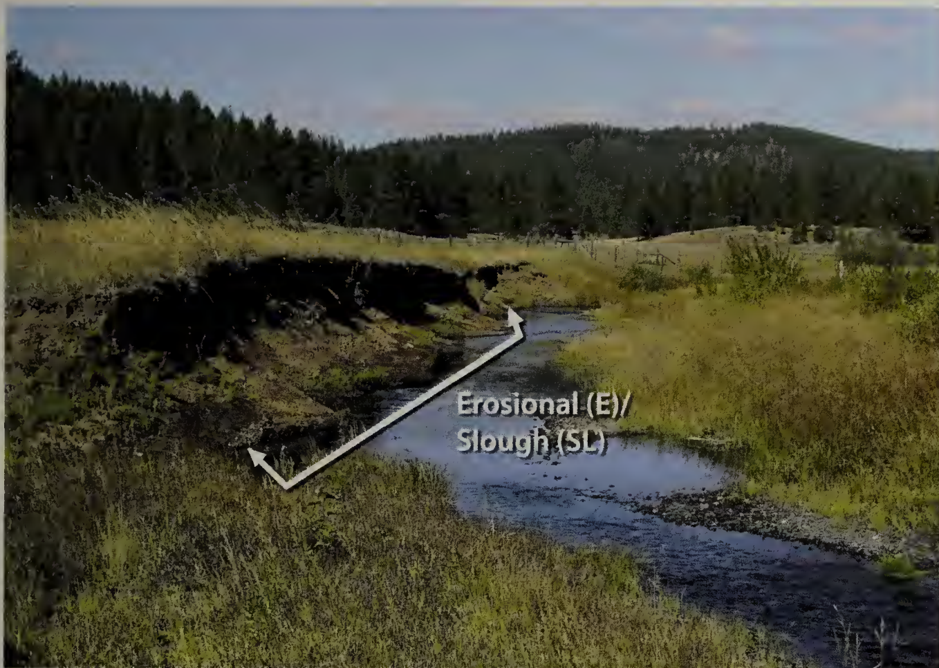
Figure 9. The streambank is erosional (E). It has a bank angle of more than 10 degrees from vertical with no bench to capture the sediment, and thus the sediment enters directly into the stream as slough (SL) (Burton et al. 2011).
