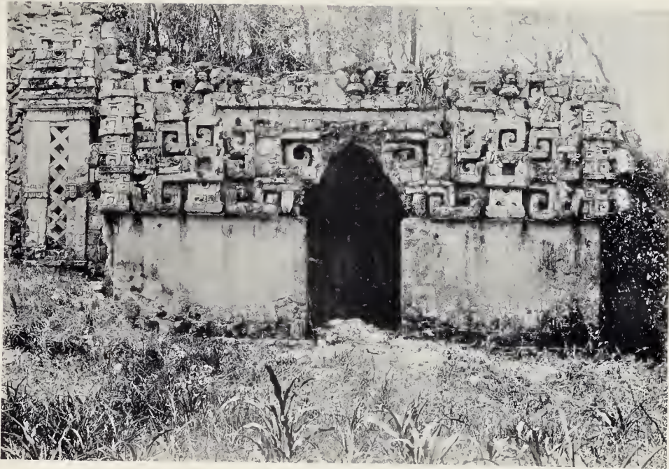
1. HICHOB. LEFT WING OF PRINCIPAL STRUCTURE. MASK PANEL OVER DOORWAY.
