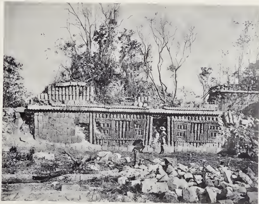
2, LABNA: BUILDING NORTH OF PORTAL: MASK PANELS IN LOWER ZONE, SHOWING SUBSTITUTION OF GEOMETRIC MOTIFS FOR THE ORIGINAL PARTS.
