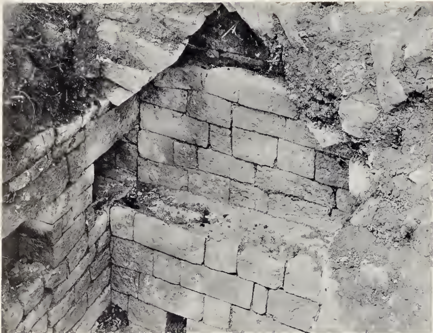
1. COPAN: SMALL VAULTED CHAMBER, SHOWING NICHE, SIDELAYS, AND ROOFING STONES.
