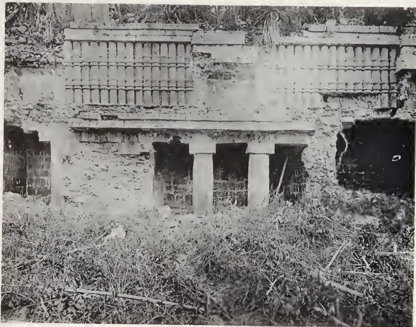
1, CHACMUTUN: EDIFICE 1, SHOWING USE OF COLUMNS FOR SUPPORT AND DECORATION, ALSO ROOF NICHS OVER DOORWAYS.
