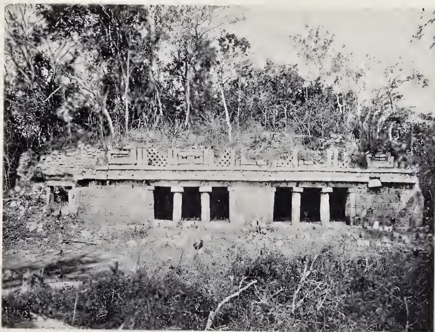
2, LABNA: PALACE, EAST WING OF UPPER RANGE: SIMPLIFIED MASK PANELS OVER WIDE DOORWAYS, FLANKED BY LATTICEWORK AND FRET PANELS.
