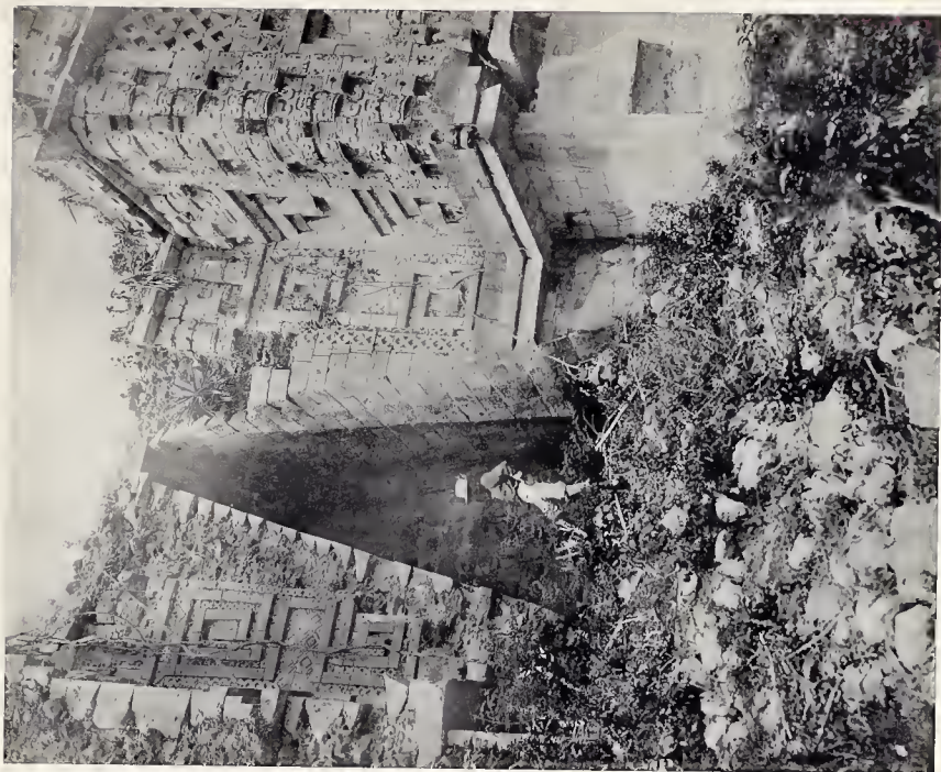
2. UXMAL: SHALLD PORTAL VAULT IN THE HOUSE OF THE GOVERNOR. THE VENER CHARACTER OF THE CUT STONE IS EVIDENT.
