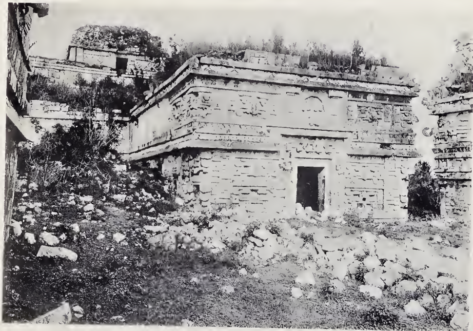
2. CHICHEN ITZA. CASA DE MONJAS: EASTERN FAÇADE OF THE EAST WING.
