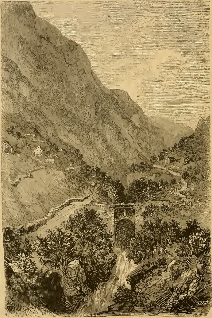
THE ARTIGUE BRIDGE AT SCIA.
