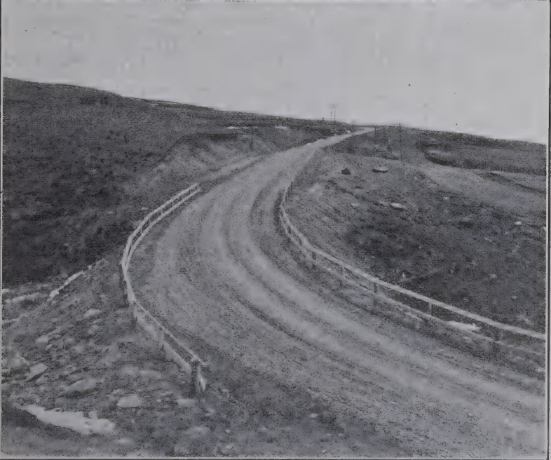
Above—Completed gravel surfacing under The Canada Highways Act on the Main Highway, near Midnapore. Below—Revised location of Main Highway near Cochrane, showing protection at curves. Abandoned road on right.
