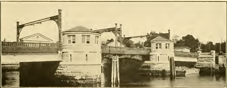
BRIDGE OVER FLUSHING CREEK AT JACKSON AVENUE
