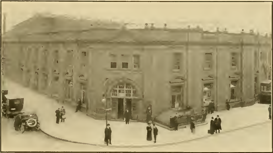
FLATBUSH AVE. STATION, BROOKLYN.
