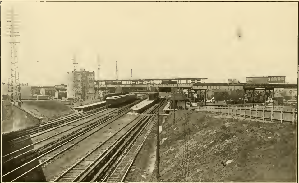
JOINT TRANSFER STATION AT WOODSIDE
