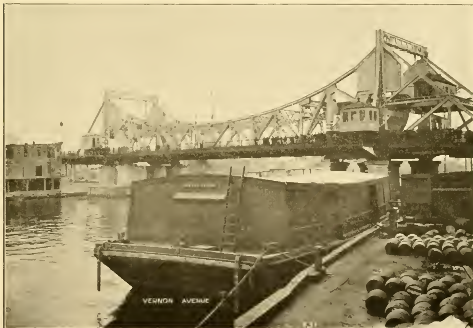
VERNON AVENUE BRIDGE OVER NEWTOWN CREEK
