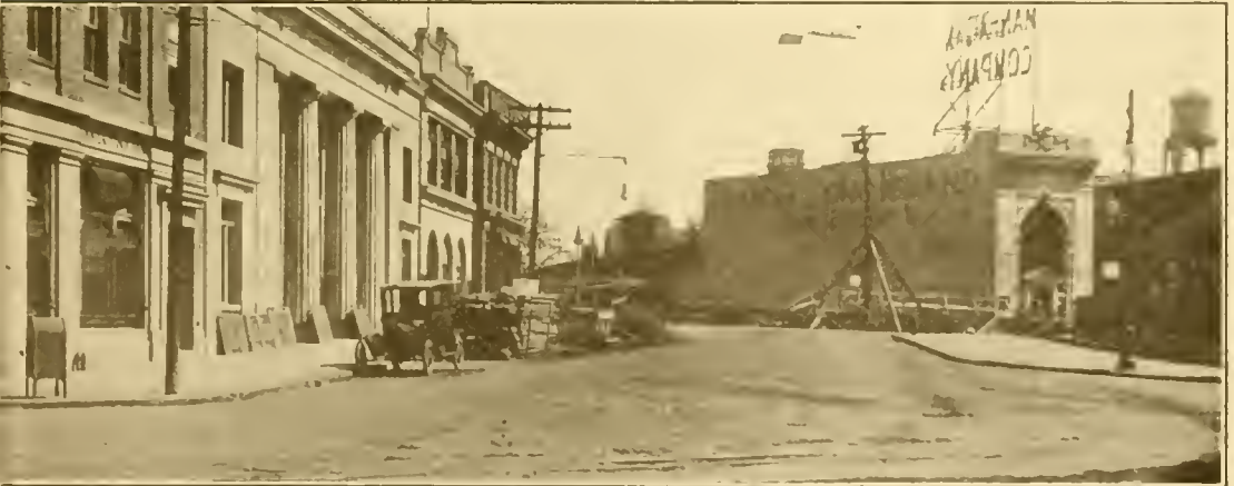
Photograph taken April 1920 shows new Long Island City Savings Bank Building, the First Mortgage Guarantee Company new building, the Title Guarantee and Trust Co. building upon which construction work had just started, and Long Island City branch of The Bank of the Manhattan Company.
