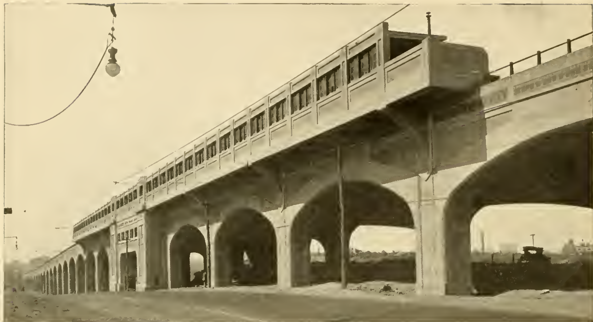
THE MASSIVE CONCRETE STRUCTURE IN THE CENTER OF QUEENS BOULEVARD, LOOKING TOWARDS THE BRIDGE PLAZA.
