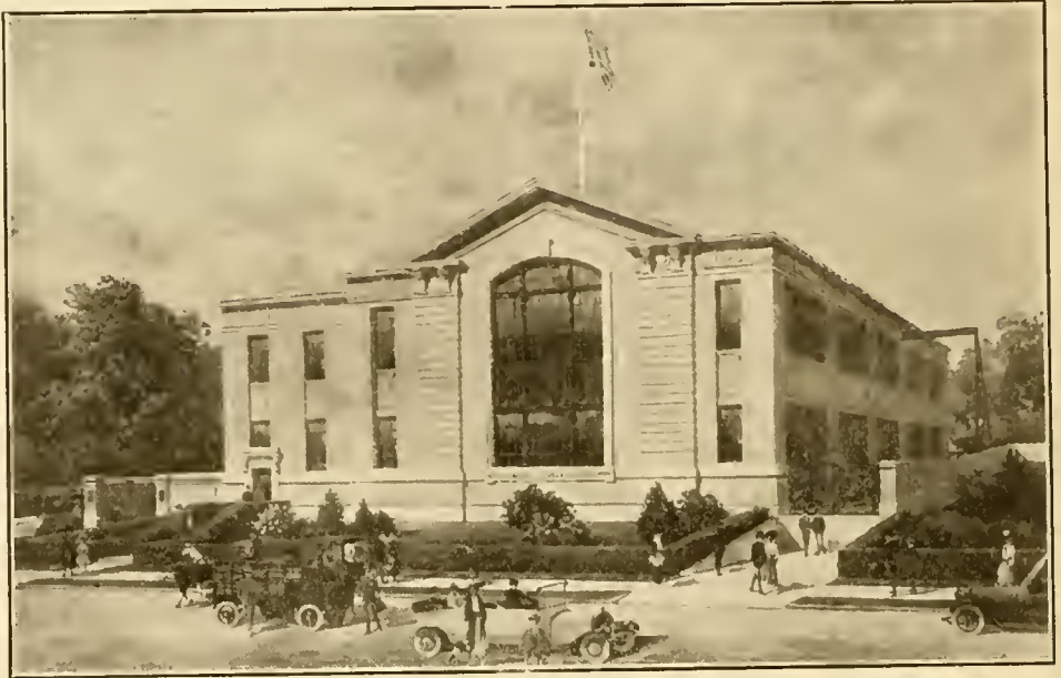
STATION No. 1—FLUSHING
