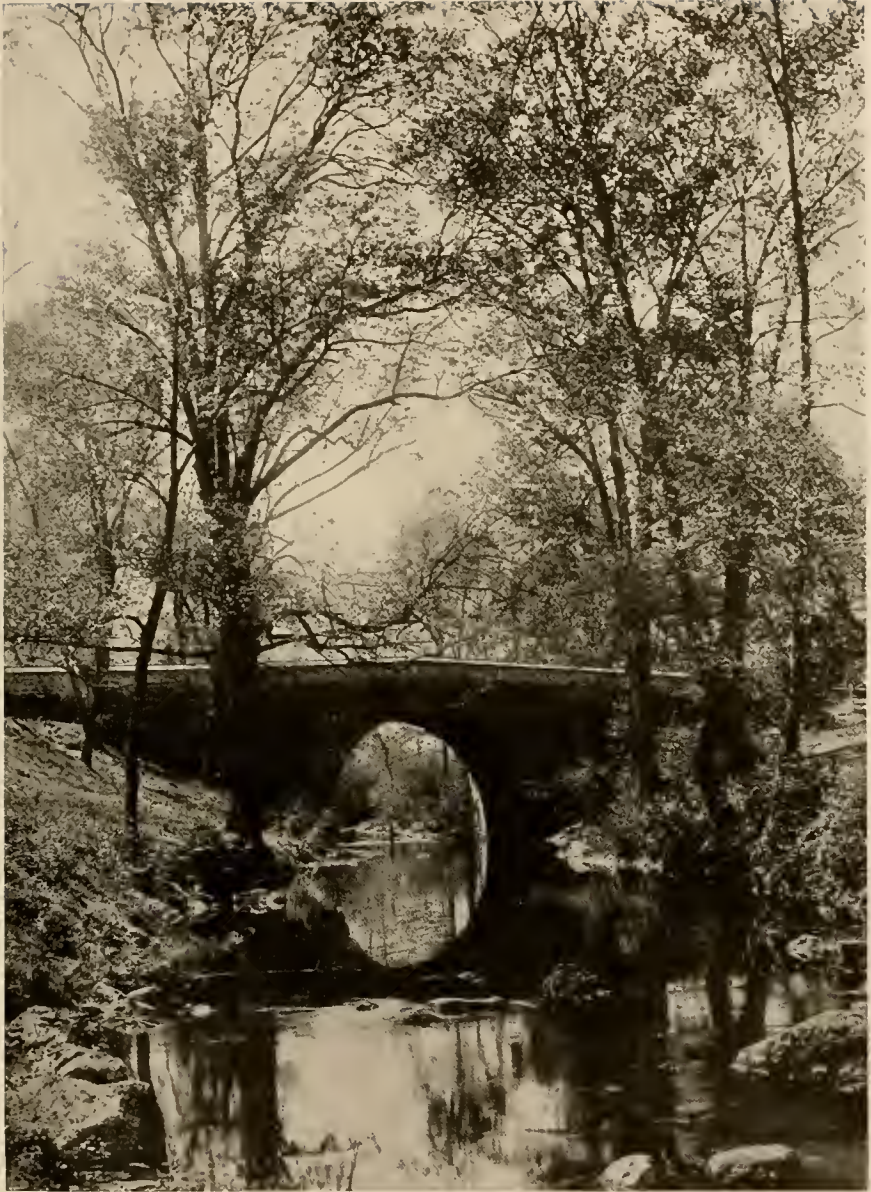
OLD BRIDGE OVER CRESHEIM CREEK.
