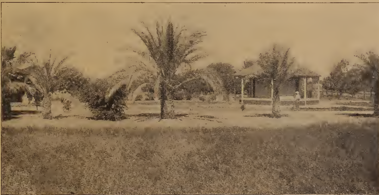
OFFICE OF THE PHOENIX SUB-STATION WITH DATE PALMS SURROUNDING IT
