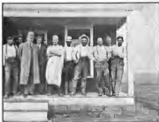
Warden Tynan and some of his convict laborers at Ranch No. 4, where one of the section gangs is quartered. One of the men in the group ran away, but came back on his own accord. Good work on the road-building enables a convict to reduce his sentence by fully one sixth
