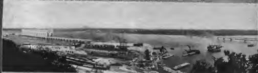
Power Plant Views
