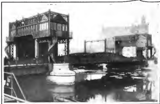
A double-leaf city bridge of the trussion type at the entrance to the port of Copenhagen, Denmark
