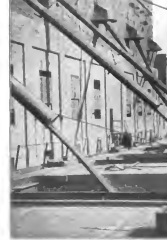
Loading lake freighter with 400,000 bushels of grain. Each of the loading spouts discharges 25,000 bushels every hour
