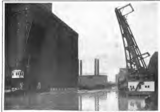
A city bridge at Puller Street, Chicago—a type of the double-leaf trussion bascule
