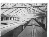
Their own Freight Sheds accommodating 40 Cars at a Time for outgoing Freight
