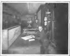
Two views of the underground switch-signal “tower” at the Grand Central Terminal, New York. On the left is shown the tower director viewed in front of the diagram of the tracks on ground level, the movement of trains being indicated therein by lights. On the right is shown the electric switch-signal system.
