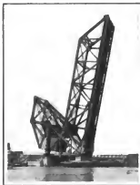
A single-leaf trussion bascule railway bridge
