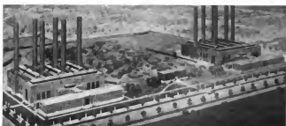
Northwest power house, Commonwealth Edison Company, Chicago, from architect's drawing. Part of the section shown at left is built and in operation with two 27,000-horsepower units.
