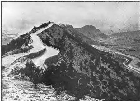
The famous "Skyline Drive" at Canon City, Colorado. This road was built by convicts from the Colorado State Penitentiary, and it is one of the most remarkable scenic highways in the world.
