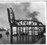
Broadway Bridge, Portland, erected at a cost of $1,600,000
