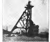
Type of Butte Skycraper, with a capacity 3000 feet deep. The picture represents the Diamond Hole with a steel head four 36 feet high. The left-hand tower in the picture is the Lamesa shaft, also one of the Anconada Copper Mining Company's properties. It is of steel construction, and is 118 feet high.
