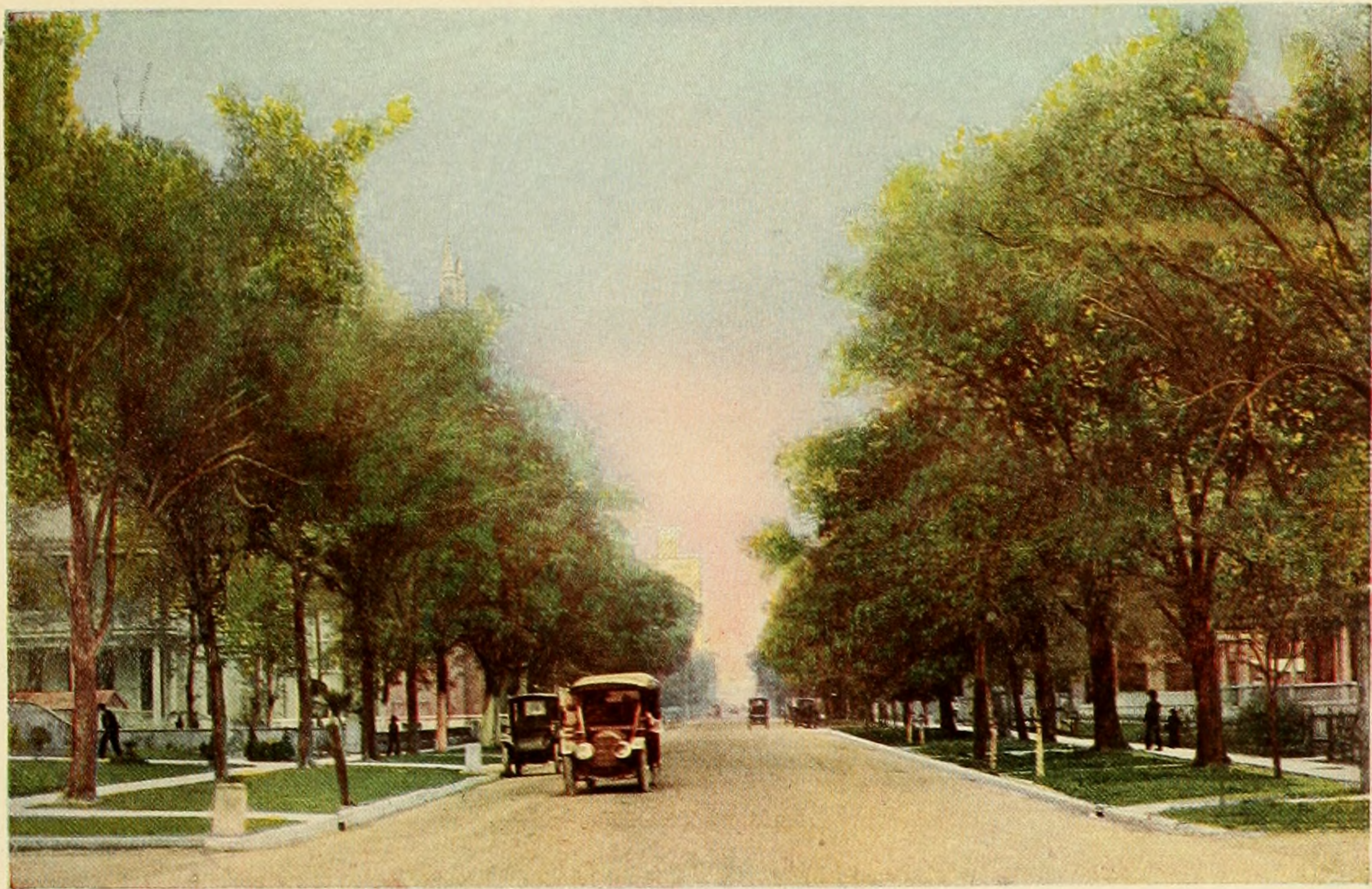
Main Street North From Bell Avenue. Houston Is Noted for Its Great Trees and Is Known as the "Magnolia City."
