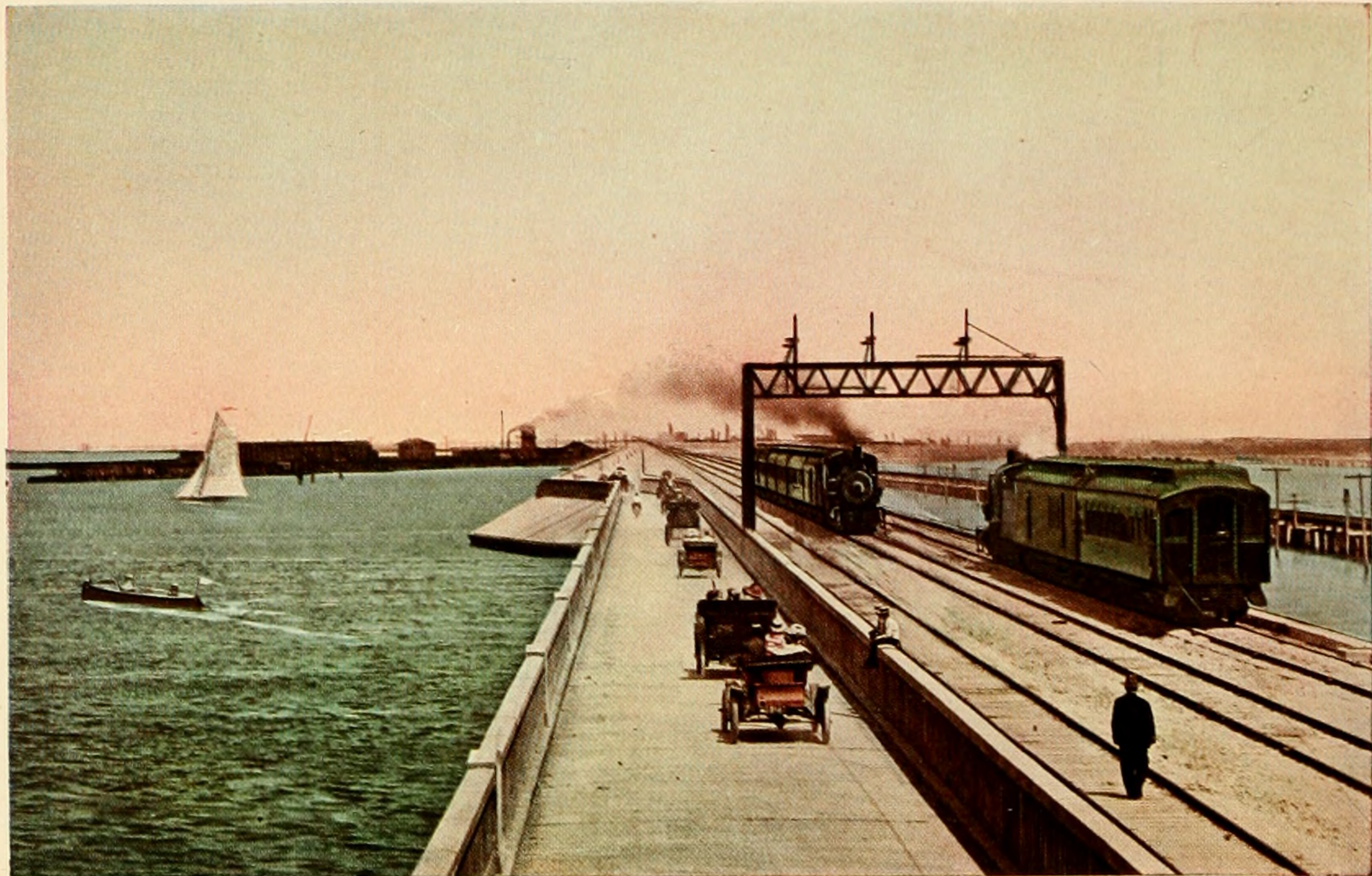
View of the Famous Causeway. Built of Reinforced Concrete. Is Two and One-Half Miles Long. Cost $2,000,000.
