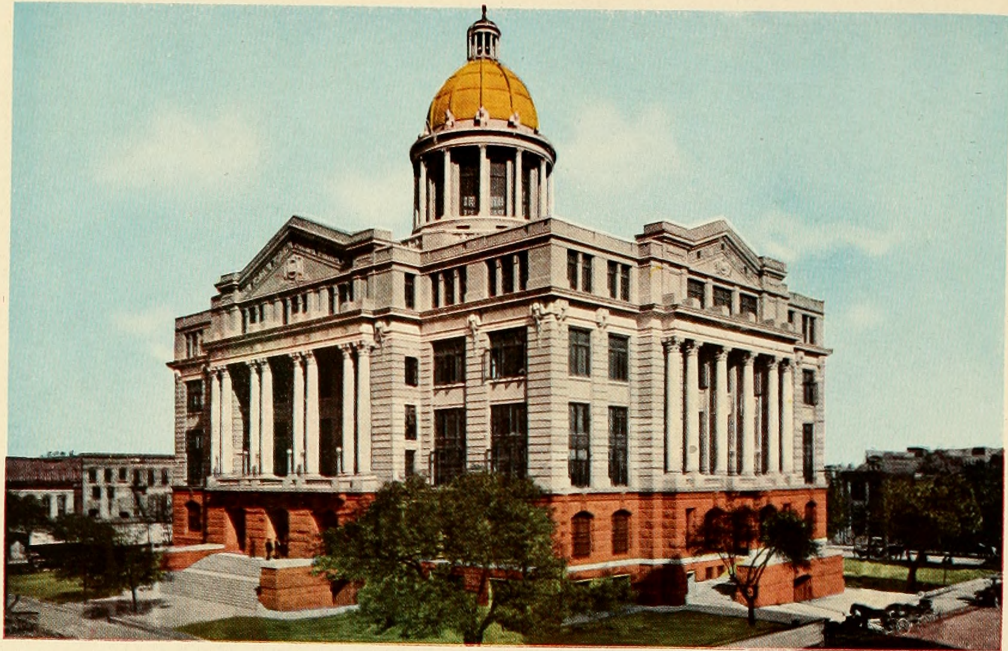
Harris County Court House at Houston. Harris County, With Taxable Valuations of $128,500,000, Is the Richest County in Texas.
