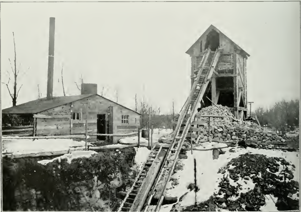
Globe Refining Company's graphite mine, near Port Elmsley; view showing shaft house.
