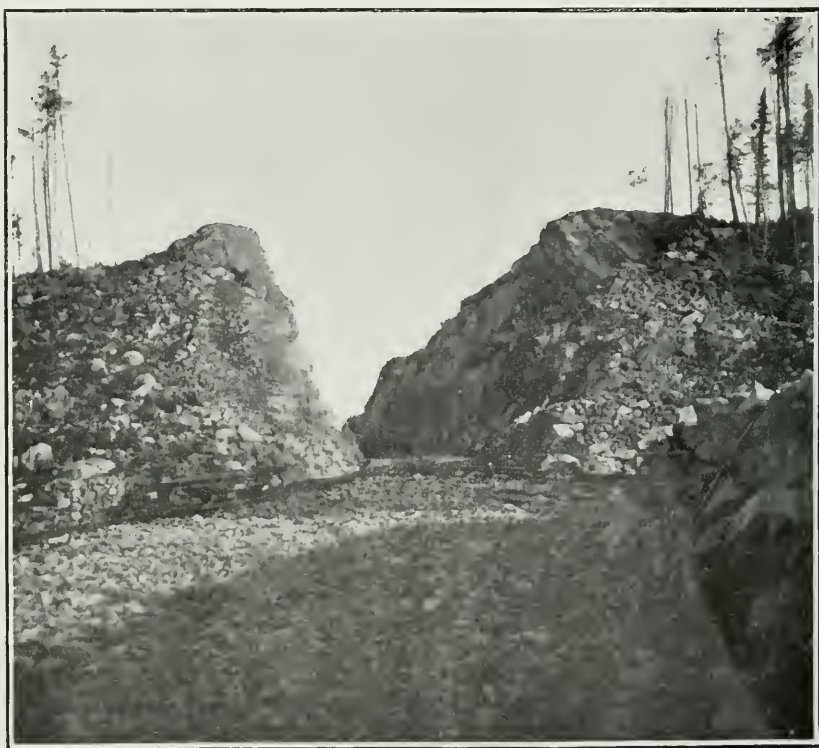
Cut 72 feet deep, Grand Trunk Pacific railway, near Vermilion pyrite mine.
