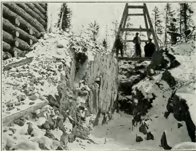
Open cut, Boyd-Gordon, shaft in back ground, April 1909.
