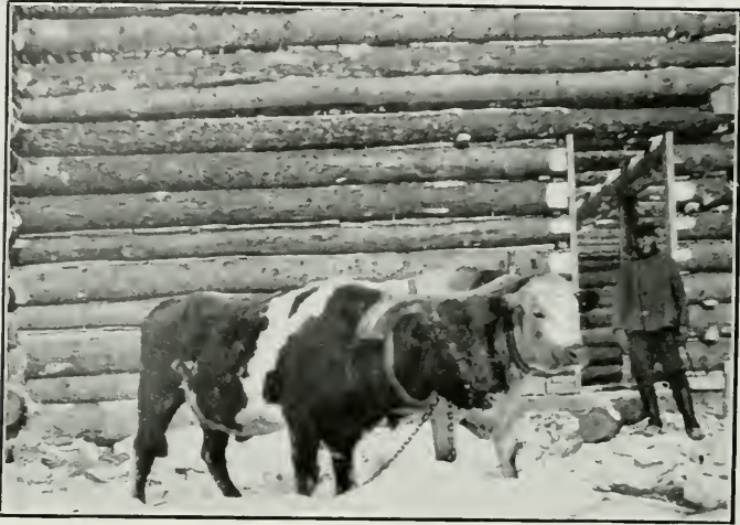
Hotel in process of construction, Gowanda, February, 1909.
