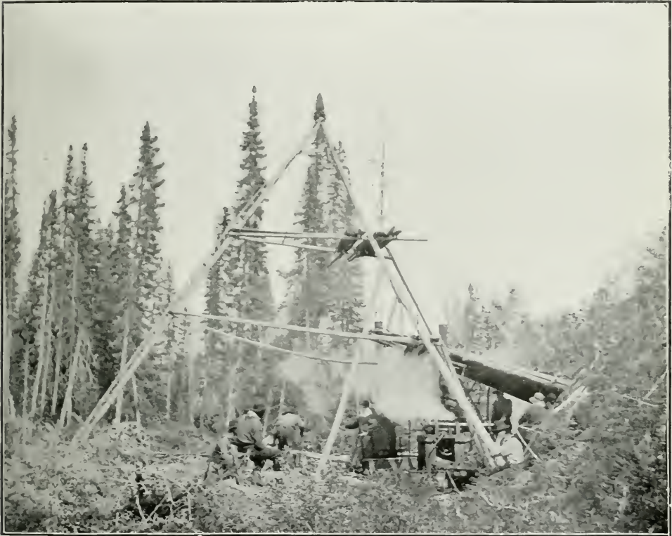
Fig. 19. Diamond drill at work on the Winter Camp claims.
