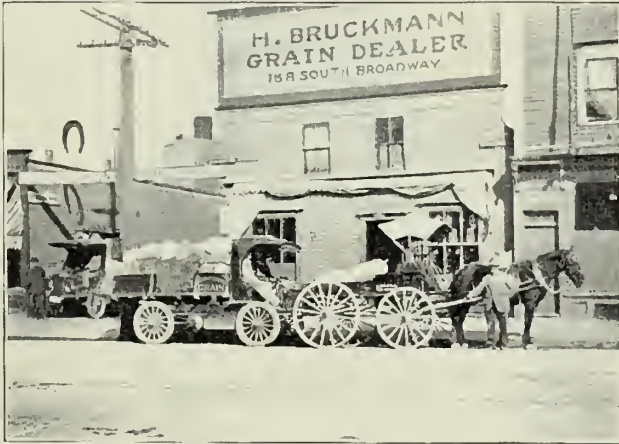
First Load out of Three that was Going to Andover that Afternoon
