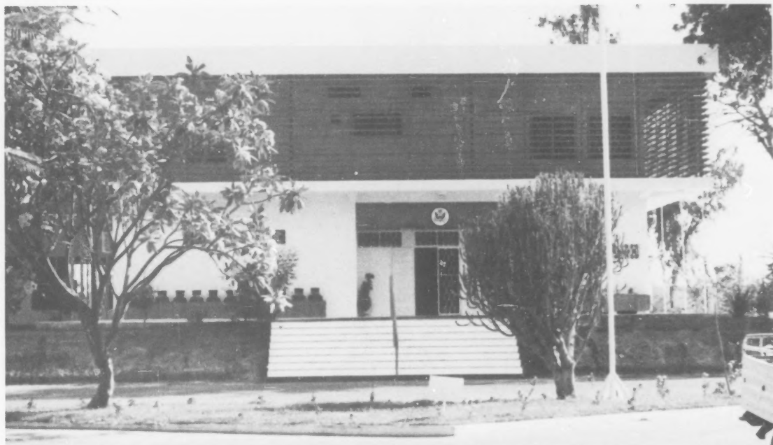
The embassy after the renovation.
