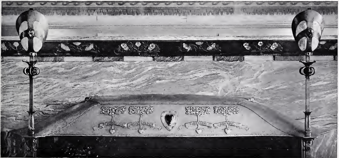
Canopy of Electric Light Carriers in Steel, Mother-of-Pearl, and Cast Ruby Glass.
