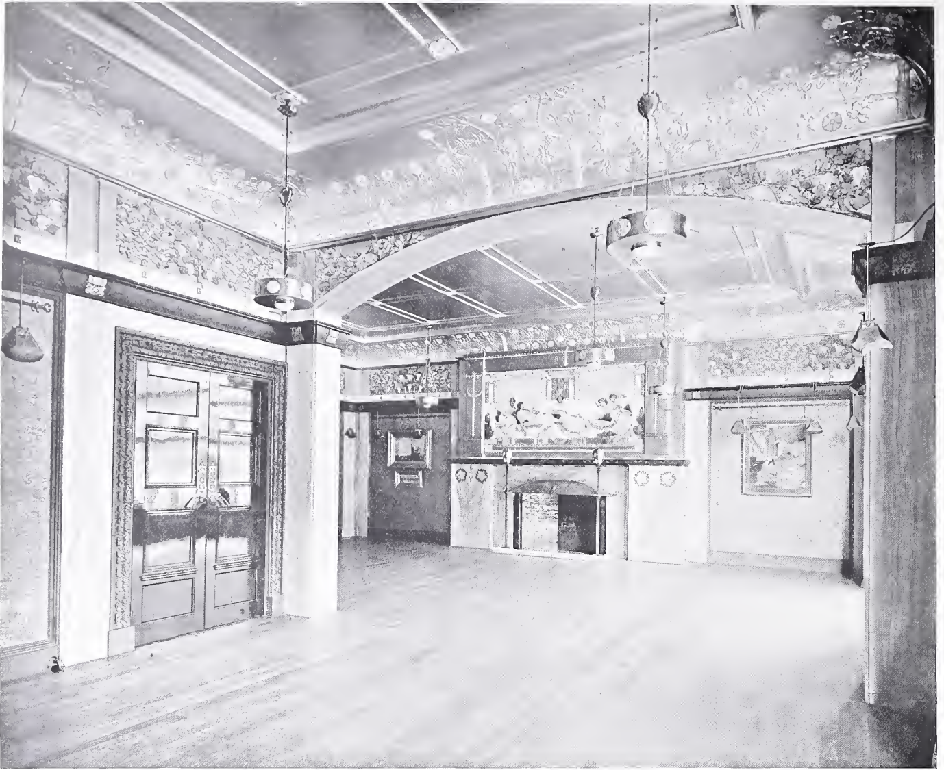
View in Room.
