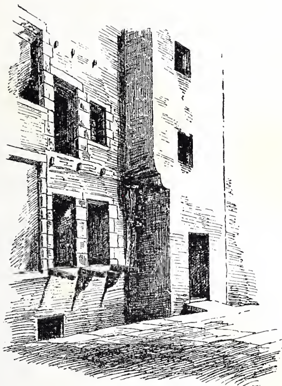
FIG. 3. TRACES OF TIMBER PROJECTION ON FACE OF OLD EDINBURGH STONE HOUSE
