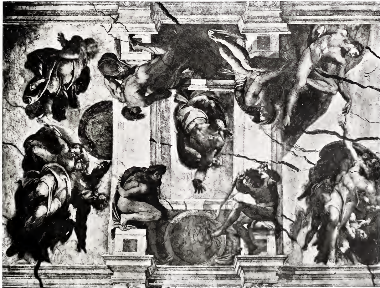
CENTRAL PORTION OF THE SISTINE CEILING, WITH THE NATURAL CRACKS MARKED IN BLACK INK
