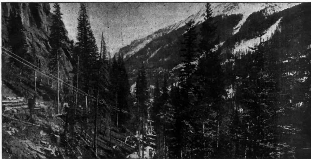
Line through the Timber.
