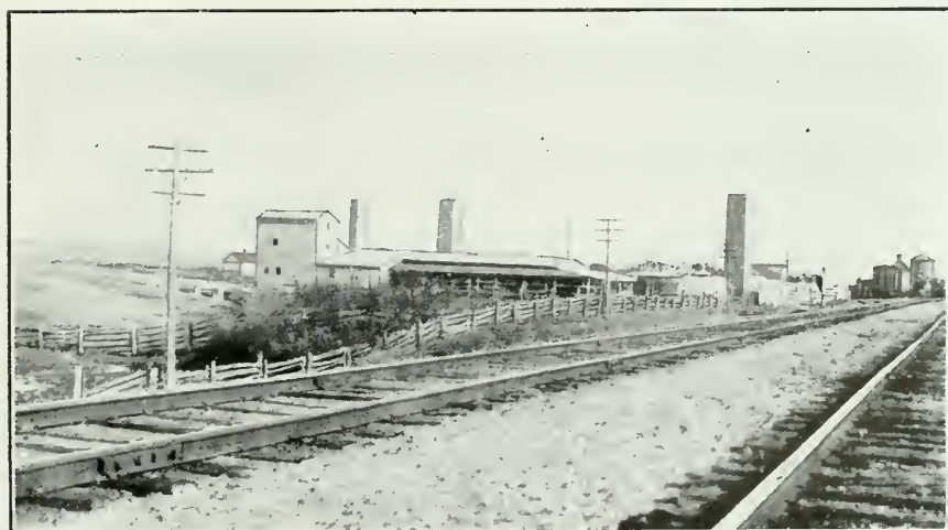
LA CIE DE TUYAUX DE DRAINAGE, LTEE.— General view of the plant at L'Islet Station
