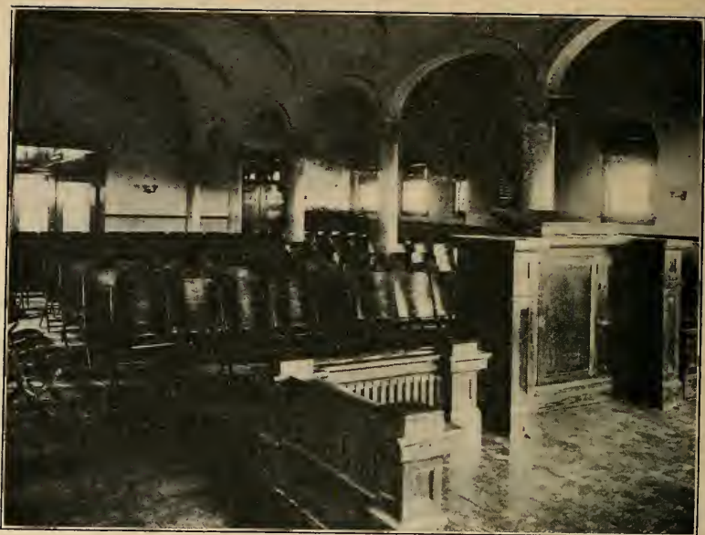
GENERAL ASSEMBLY ROOM, FOURTH FLOOR BISHOP'S BUILDING
