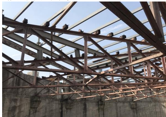
屋架為普拉特桁架 (PRATT TRUSS)
