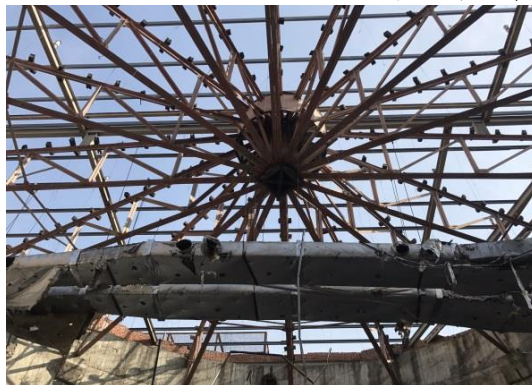
屋架為普拉特桁架 (PRATT TRUSS)
