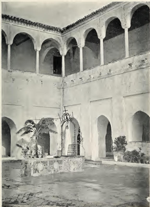
Fig. 5.— Convento de la Luz (No. 1). Copto-Arabic arches of the Central Court with fifteenth-century arcades above.
