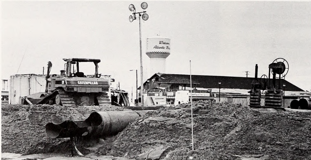
Dredge spoil disposal setup at The Circle.
