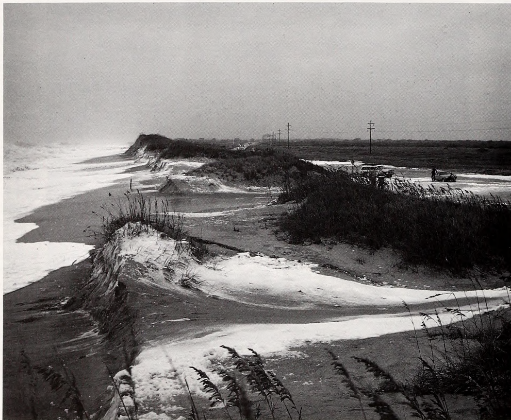
Overwash on Highway 12 at Rodanthe.
