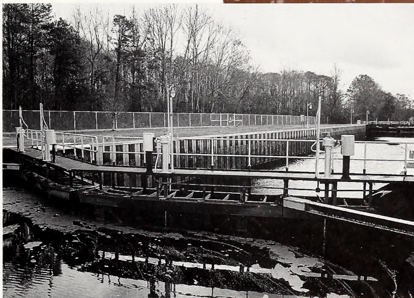
The Feeder Ditch
