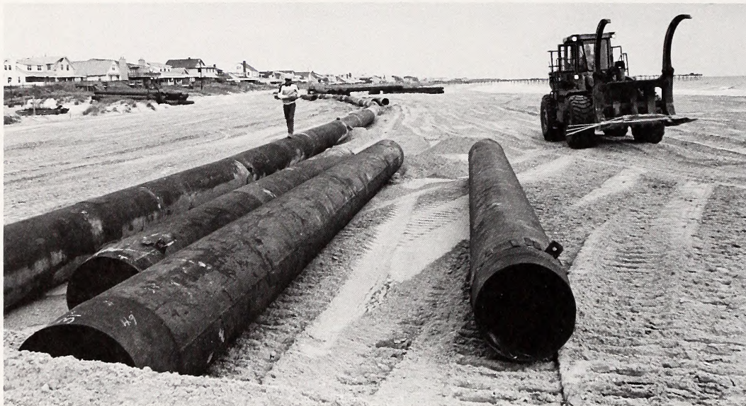
Pipes feed a slurry to Bogue Banks.
