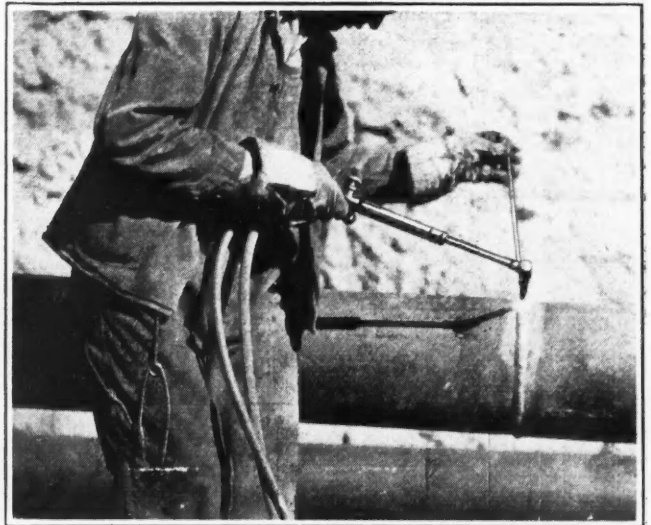
Fig. 3—Welding a joint
