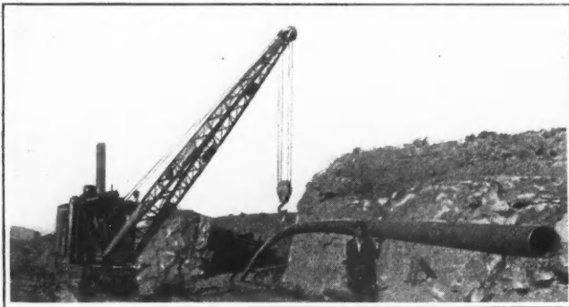
Fig. 2—Handling welded pipe line by locomotive crane
