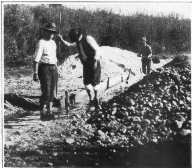
Fig. 2—As the water flows through the canal the remaining fine gravel is gently stirred with the feet
