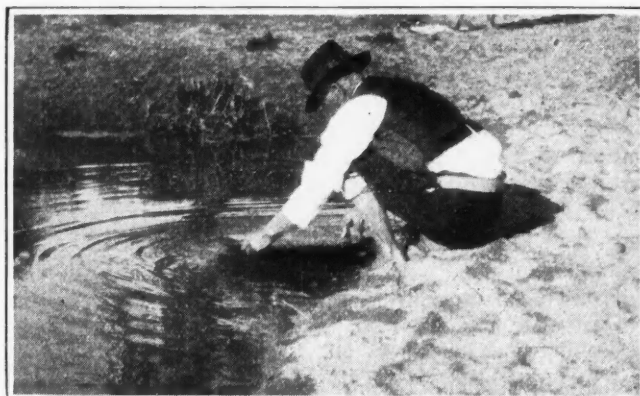
Fig. 4—Final washing is done by panning with a batea
