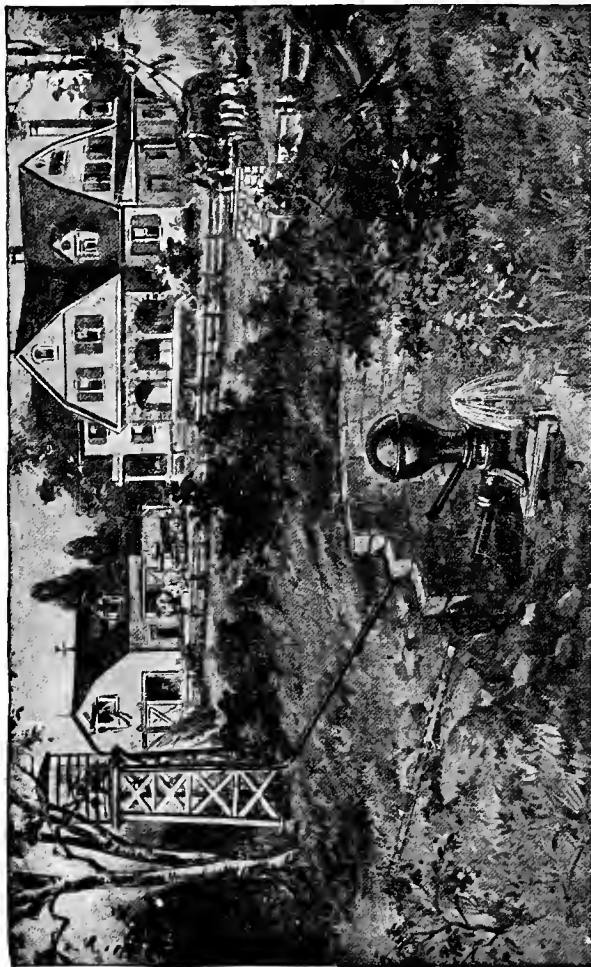
Fig. 78. Hydraulic ram at work.
