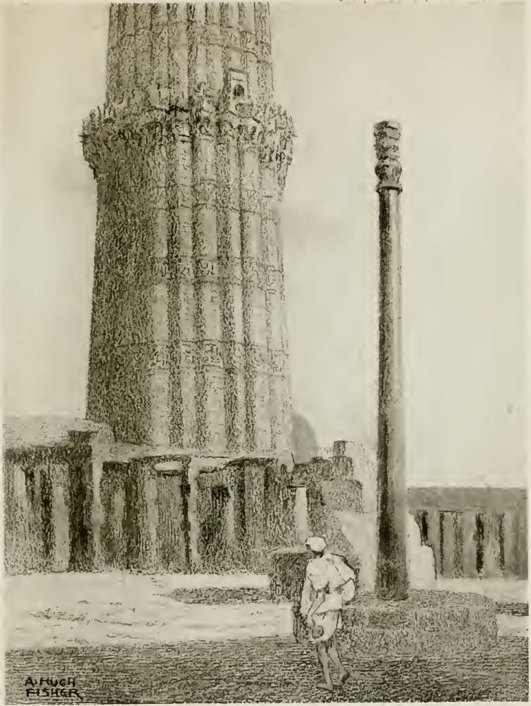
THE ROSE-COLOURED GRANITE TOWER
