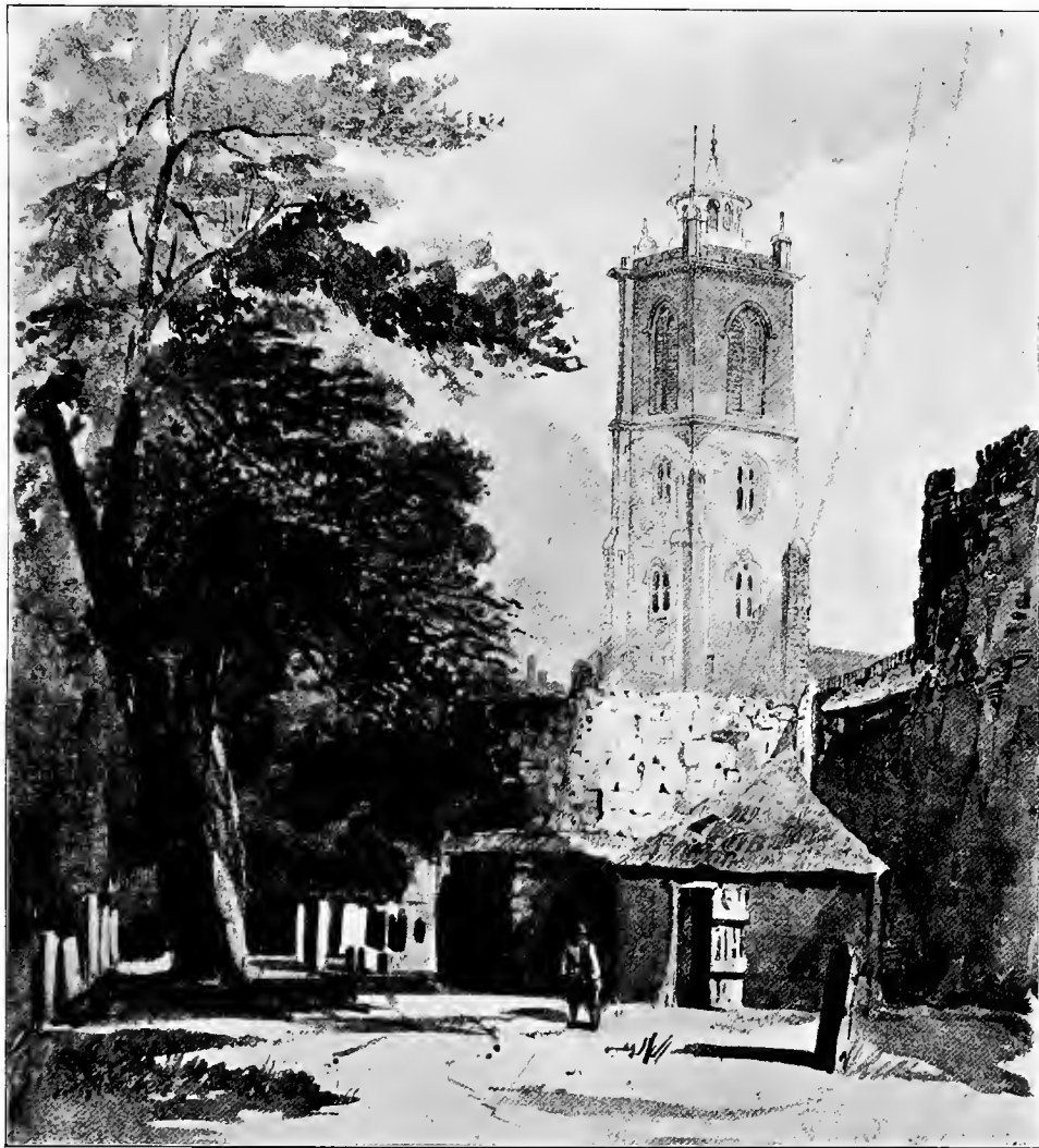
BASTION OF THE CITY WALL, IN THE CHURCHYARD OF ST. GILES'S, CRIPPLEGATE.
