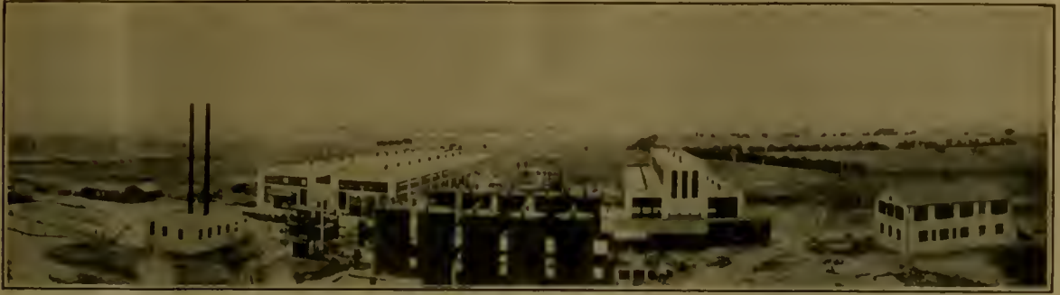
FIG. 1.—Helium production plant, Fort Worth, Texas, operating at the present time.
