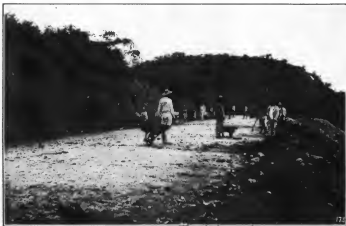
BUILDING A NEW WAGON ROAD NEAR SABANA GRANDE, HONDURAS.
