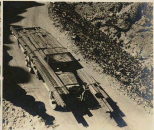
50-ton truck hauling reinforcement steel
