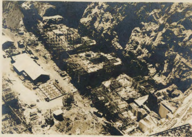
Nevada wing view downstream July 21
