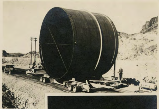
Transporting 30 foot pipe by trailer
