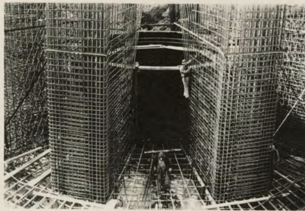
Reinforcement steel at tower base
