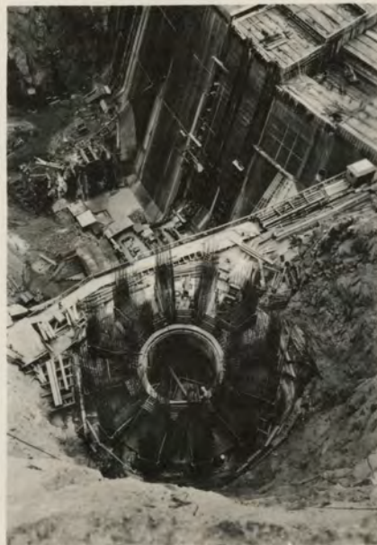
Reinforcement steel at tower base
