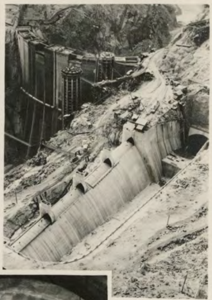
Nevada Spillway, December 10
