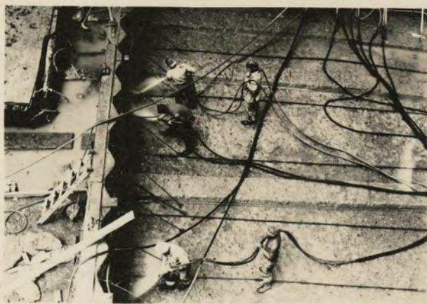
Cleaning concrete by jetting
