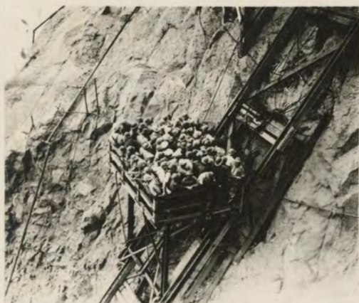
Monkey Slide on Nevada abutment
