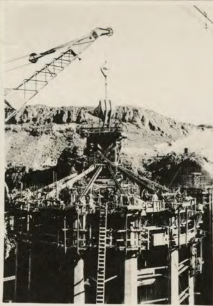
Pouring Nevada D. S. Tower October 29
