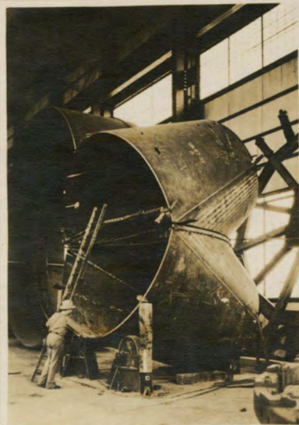
Y section for outlet pipes
