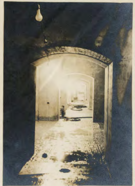
Arches in Pump gallery, Arizona wing
