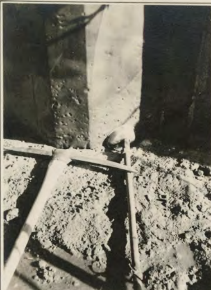
Cooling pipe installation at contraction joint
