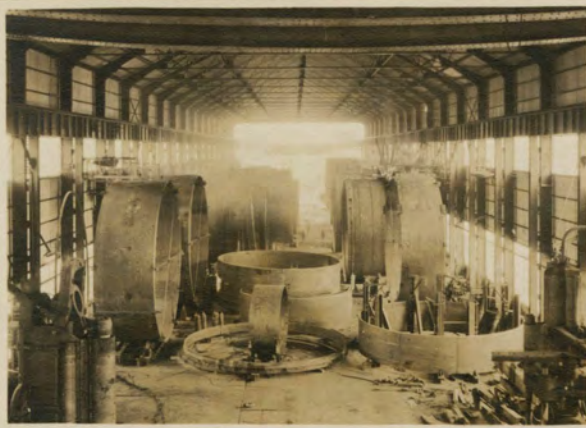
Interior of Fabrication Plant
