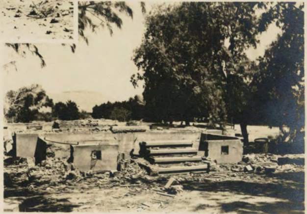
Abandoned and dismantled homesite
