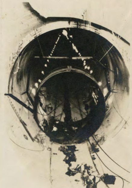
30 foot Pipe in No. 3 Tunnel
