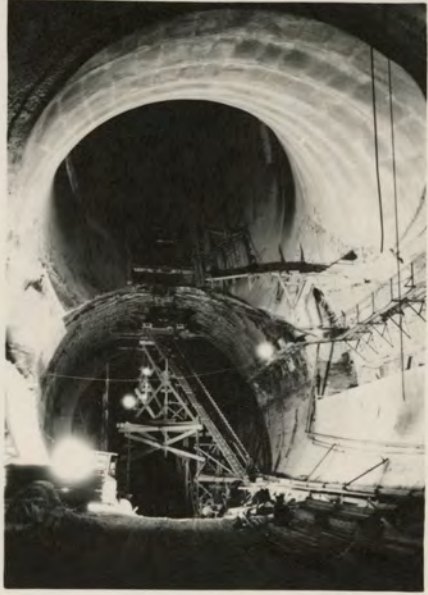
Intersection Nevada incline and Tunnel 1
