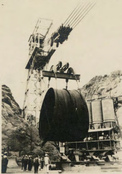
Government cableway handling 30 foot pipe
