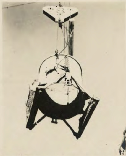
Transportation from high level concrete plant
