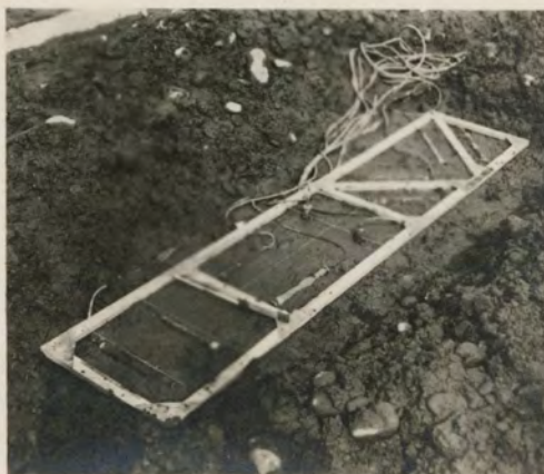
Strain meter installation and form
