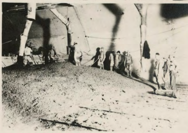
Placing concrete in U. S. Plug Tunnel No. 2
