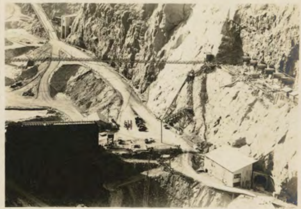
Nevada valve house and adjacent features
