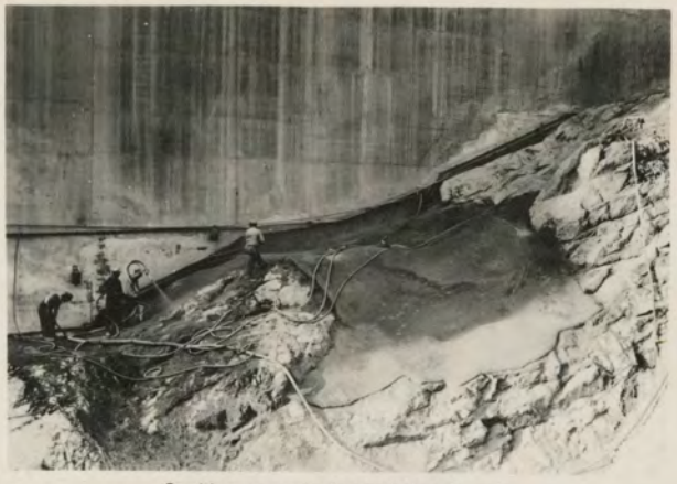
Guniting apron in front of Nevada weir
