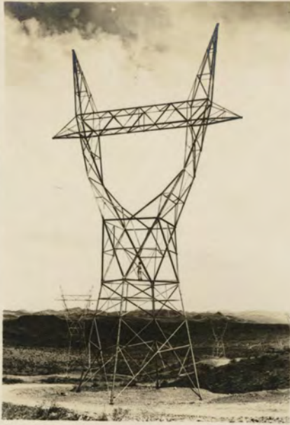
Transmission line tower of Los Angeles Bureau of Power and light
