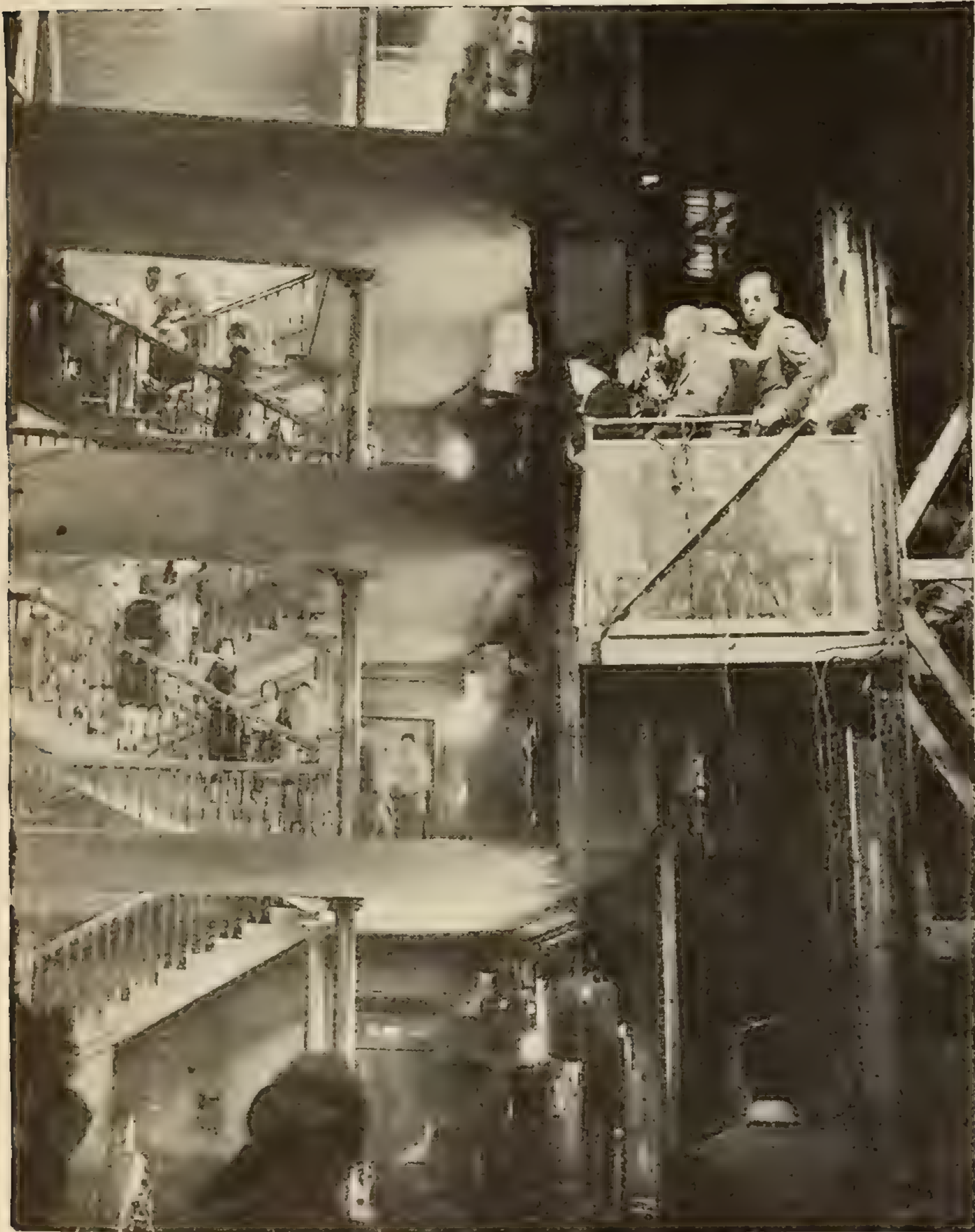
ⒸTraveling elevator cage designed by Peverell Marley for photographing scenes in 'The Godless Girl.'
