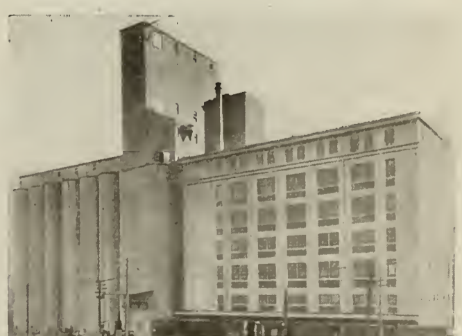
PILLSBURY FLOUR MILLS CO., MILL & ELEVATOR Atchison, Kans.
