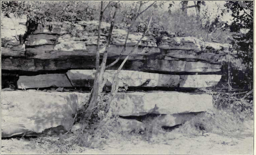
B.—An exposure of the Maxville limestone in Jonathan Creek opposite the Fultonham Depot, showing the conspicuous stratification of the upper half, due in part to solution along the bedding planes and in part to the removal of the shaly partings.
