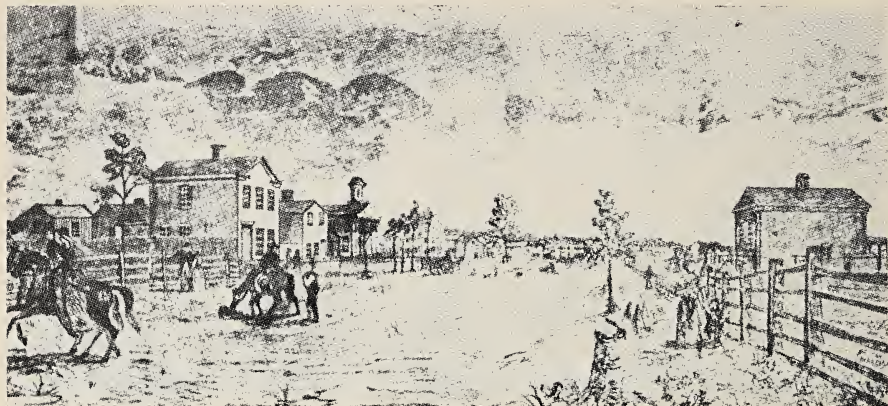
FIGURE 1. Corner of Seventh and Main Streets, Racine, in 1841 (drawing reproduced courtesy the Racine County Historical Museum).
