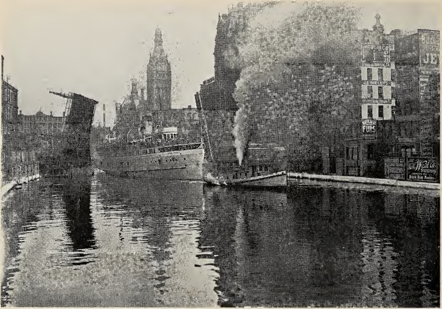
FIGURE 4. Excursion boat on Milwaukee River at Wisconsin Avenue bridge. Milwaukee City Hall in background. Marine National Exchange Bank has replaced buildings on the right. Circa 1920. (Milwaukee Public Museum photo.)
