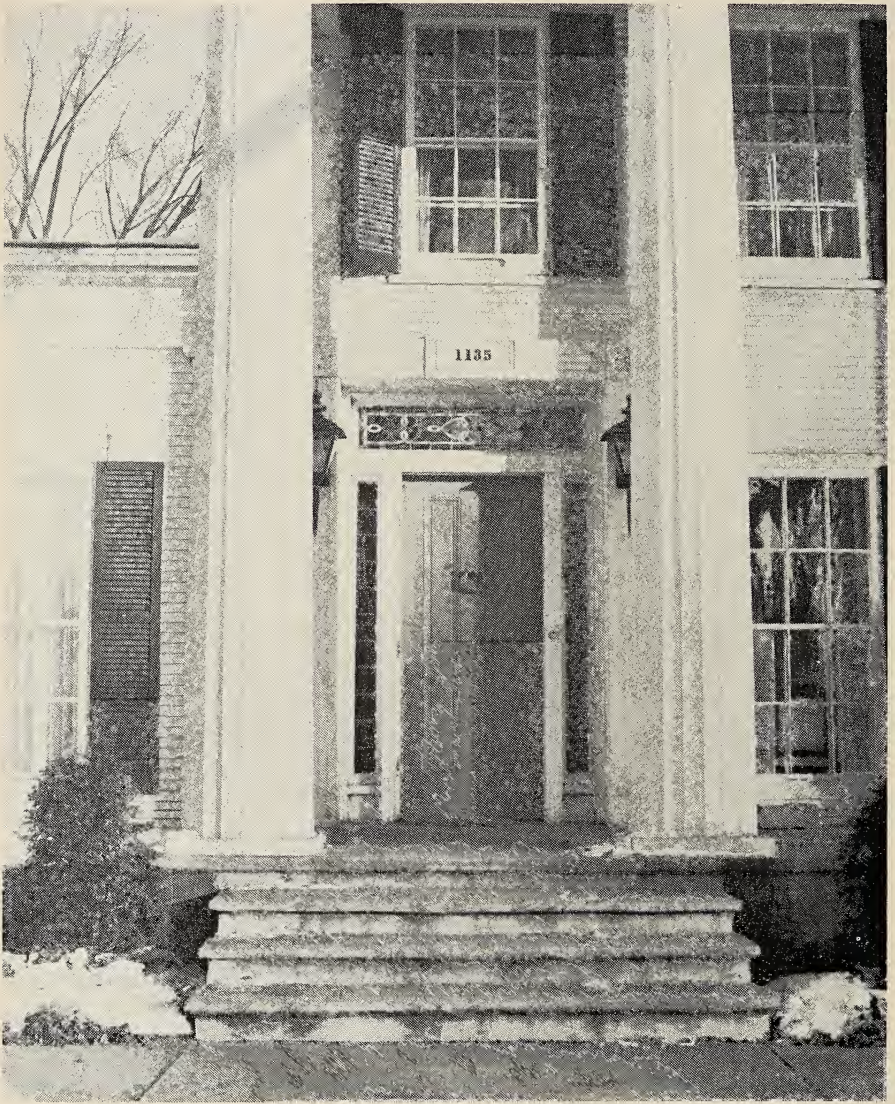
FIGURE 10. 1135 South Main Street, detail, entrance (photograph by Todd Dahlen and Peter Vallone).
