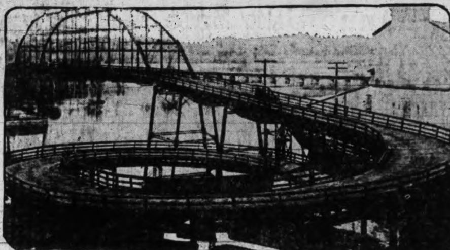
LOOKS LIKE ROLLER COASTER? GUESS AGAIN.—Hastings, Minn., city officials solved the problem of eliminating a long bridge approach from the Mississippi River into the business section. They made the terminal of the span a spiral. The bridge is an engineering freak in the northwest.
