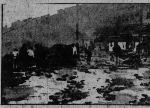
WRATH OF FIRE AND FLOOD.—The central part of Hot Springs, Ark., looked like this after recent flood waters had receded and fire was under control. No lives were reported lost, but property damage of $2,000,000 was caused.
