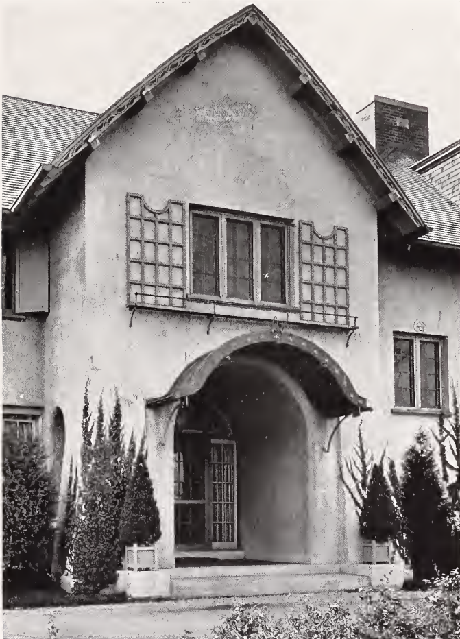
THE FRONT ENTRANCE WITH UNUSUAL GABLE
