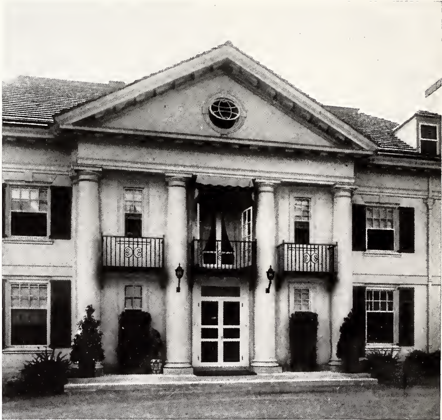
THE ENTRANCE IS CROWNED BY A STATELY PEDIMENT
