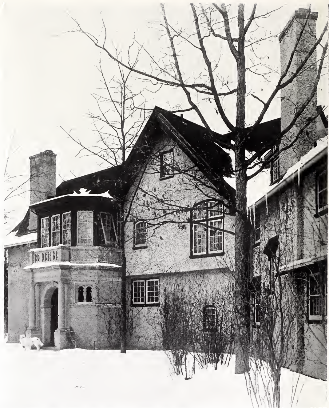
DETAIL OF ENTRANCE PORCH AND BAY SHOWING GABLES AND CHIMNEYS It is a substantial house embodying certain characteristic details of the Elizabethan period
