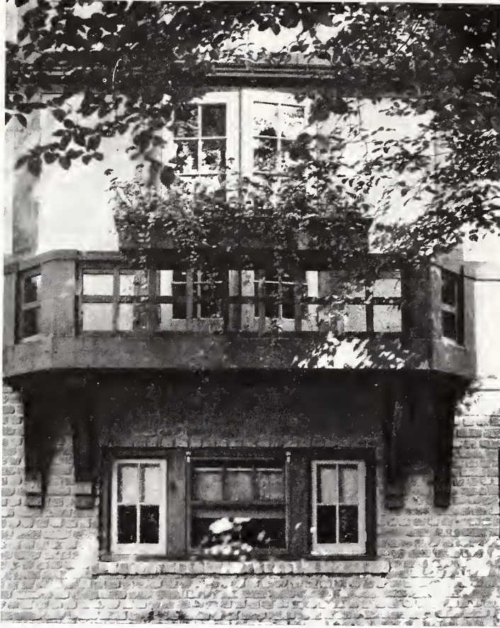
SOME BALCONIES ARE VERY SUBSTANTIAL
