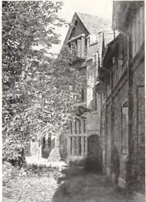
ANOTHER VIEW OF SERVICE TOWER
