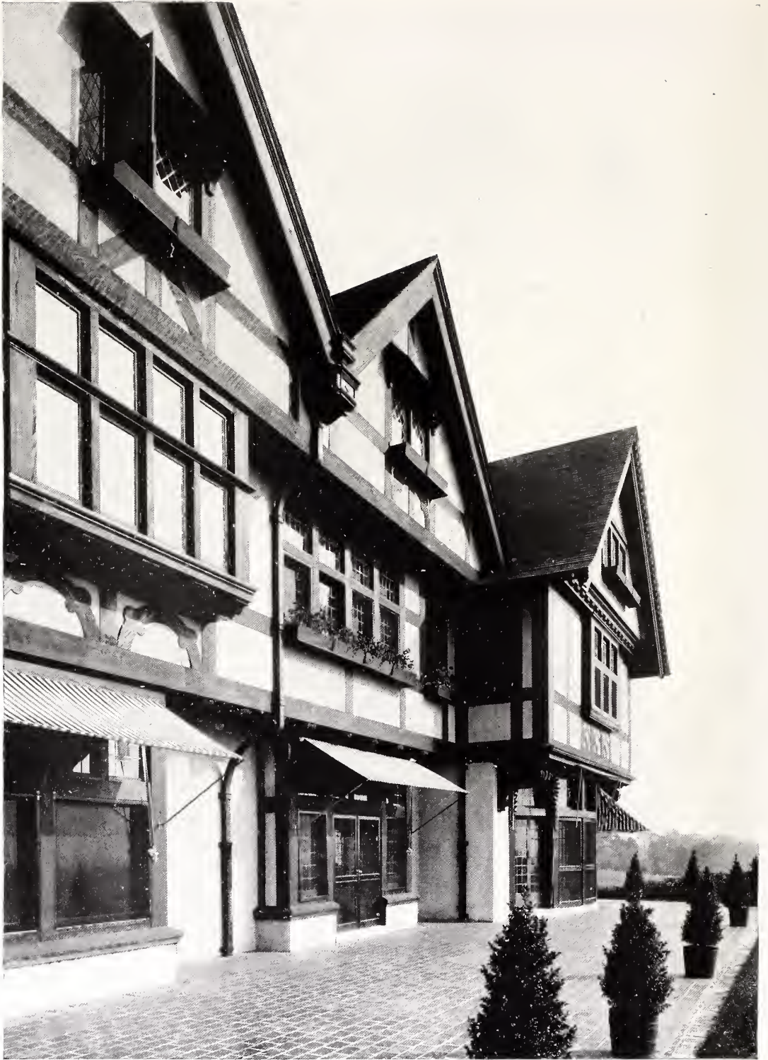
FACING LONG ISLAND SOUND IS A WIDE PAVEMENT OF RED BRICK Picturesque is this elevation with its overhanging, half-timbered gabling and projecting bays
