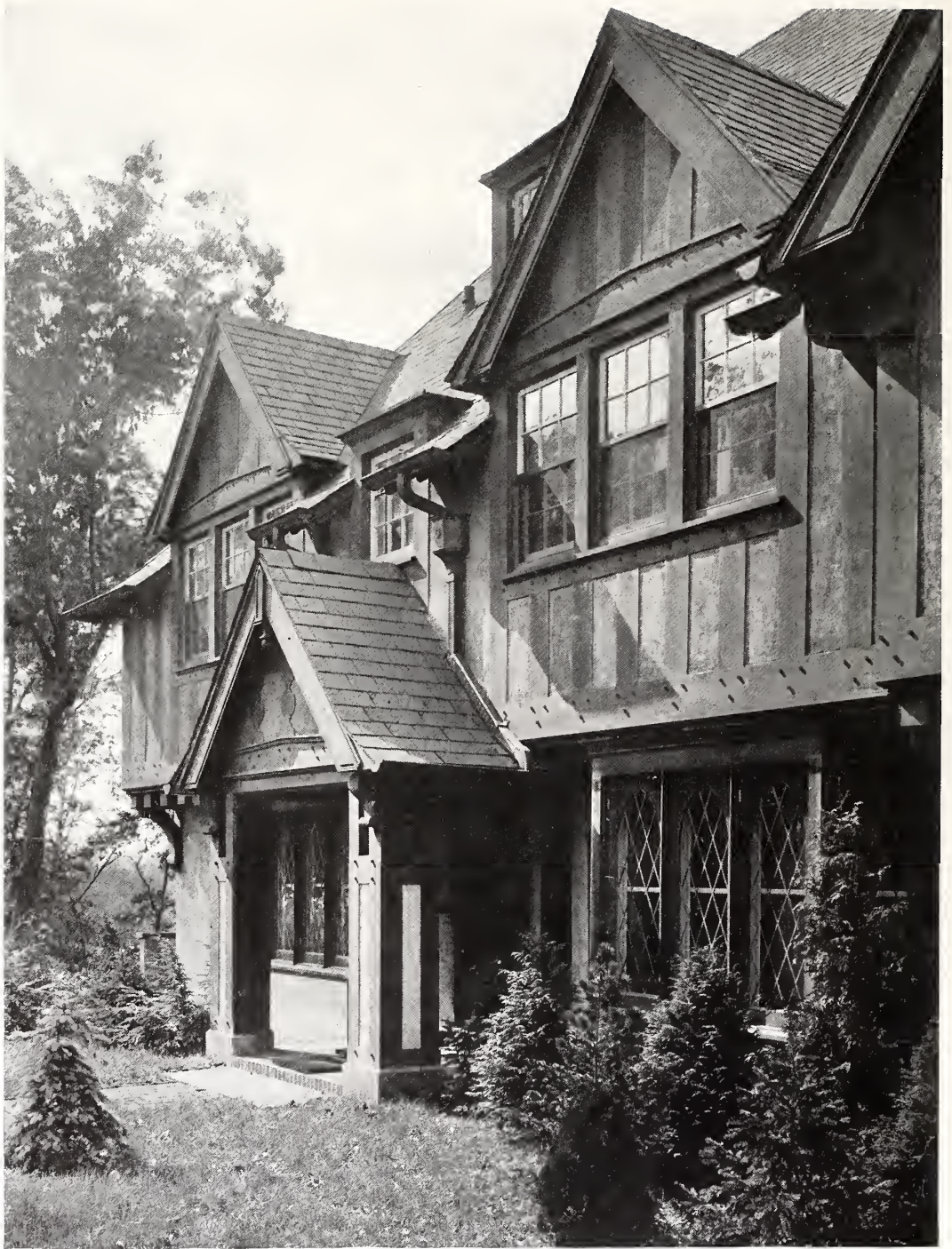
A PICTURESQUE REMINDER OF THE HALF-TIMBER METHOD OF CONSTRUCTION In an ingenious fashion the architect has permitted the upper floors to overhang. ( See page 281 )
