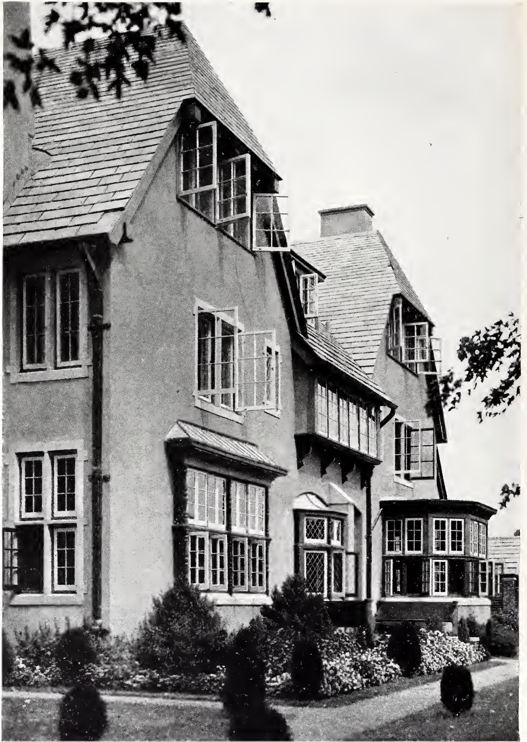
ARCHITECTURE IS SAID TO BE THE RIGHT TREATMENT OF OPENINGS In delightful variation is this interesting study in oriels and bays. Look at the wealth of casements
